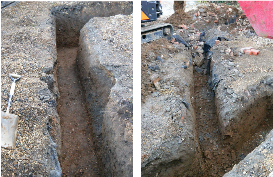
Photographs 1-2 Foundation trench, looking SE and drainage trench, looking NE
