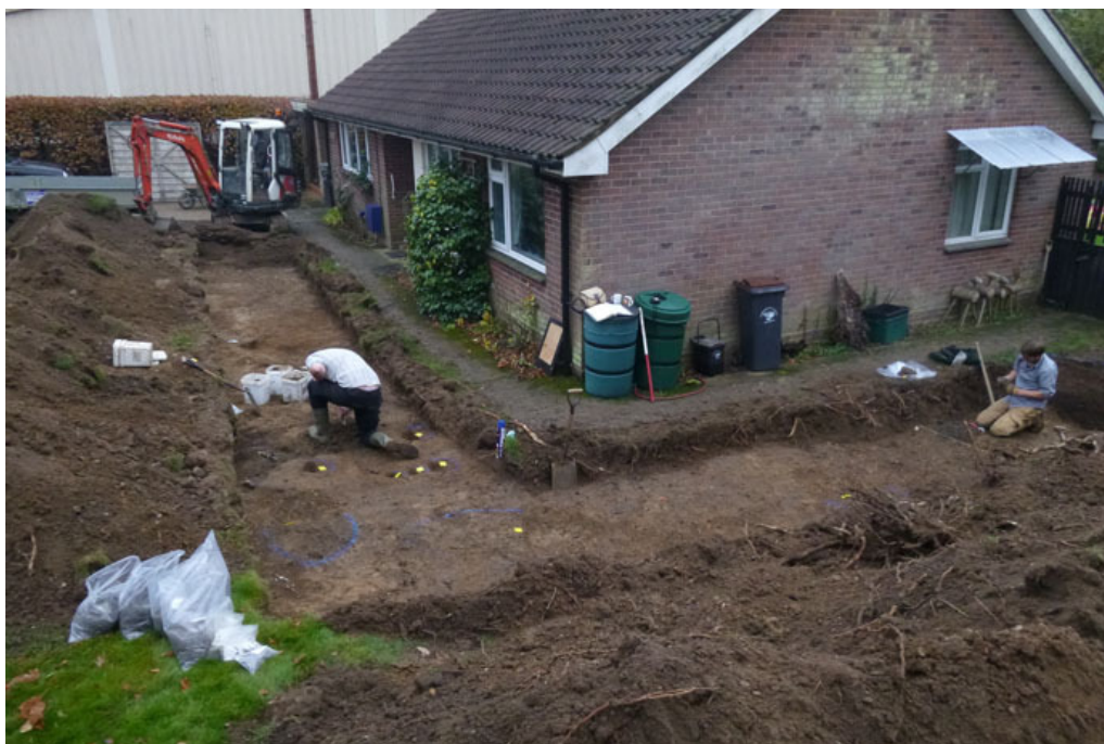
Photograph 1 Site shot, looking SE
