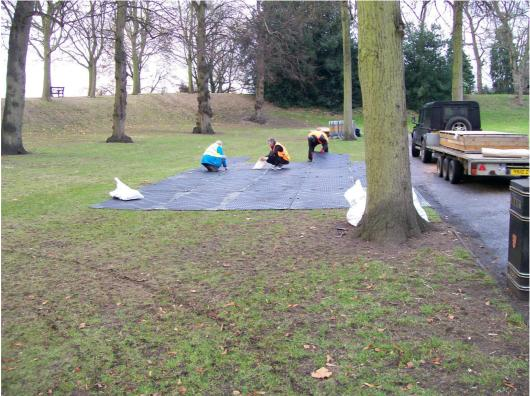
Photograph 9 Construction of matting for catering facilities, north side of Castle, looking E
