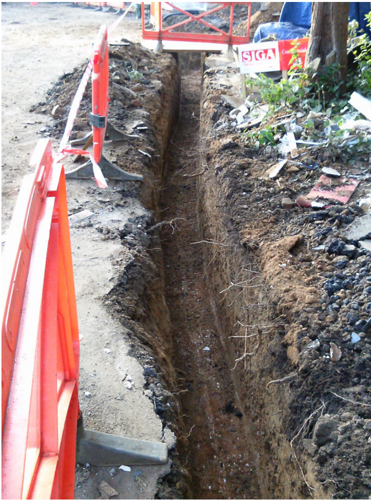
Photograph 3 Service trench, looking SW
