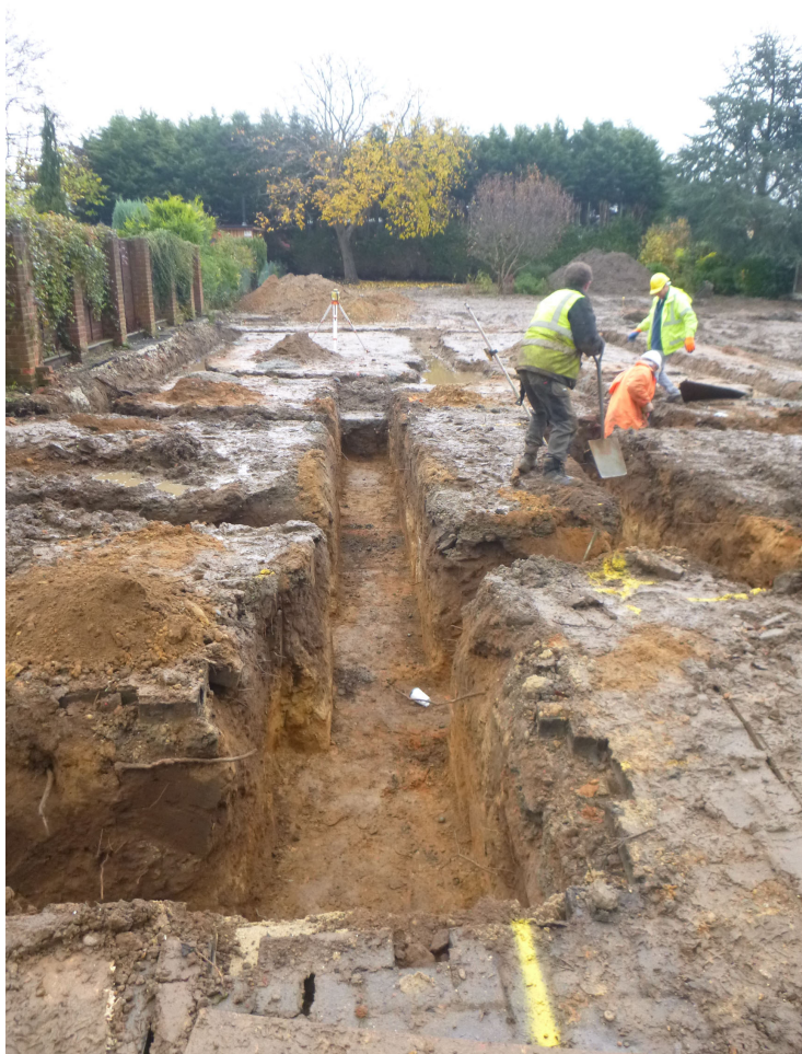
Photograph 1 Excavation of foundation trenches, looking E
