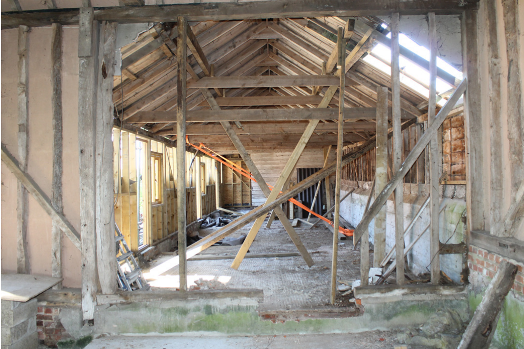
Photograph 7 Interior shot of Building B, showing supporting timbers and straps. In foreground is the northern elevation of Bay 4 (in the barn), with multiple missing studs and modern replacements. Photograph taken facing north.
