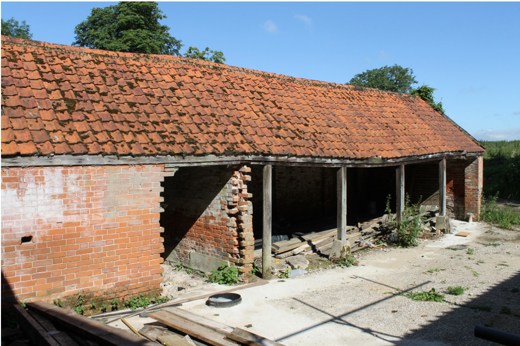
Photograph 2 East elevation of Building A – photograph taken facing north-west.
