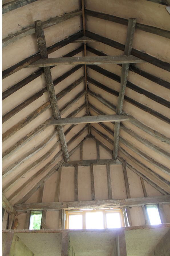
Photograph 13 Detail of midstrey's roof, showing modern purlins and collars as well as ?fire-damaged rafters. Photograph taken facing south.
