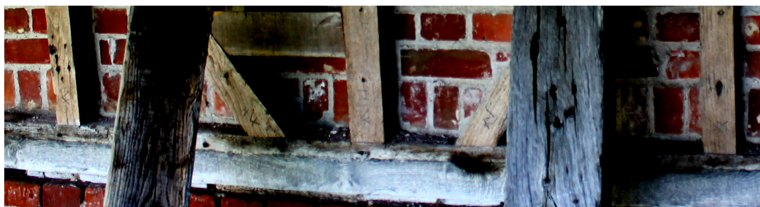
Photograph 22 Carpenter's mark visible on the exterior of studs and braces in southern elevation of Bay 2. Contrast enhanced for better visibility. Photograph taken facing north.
