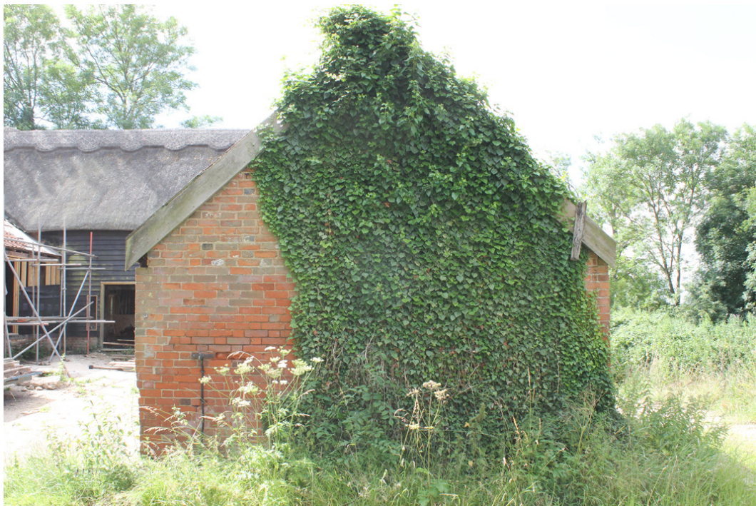
Photograph 4 North elevation of Building A, with changes in brickwork bonding visible – photograph taken facing south.
