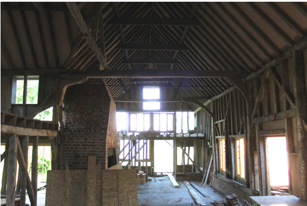
Photograph 8 Interior shot of barn – photograph taken facing west.
