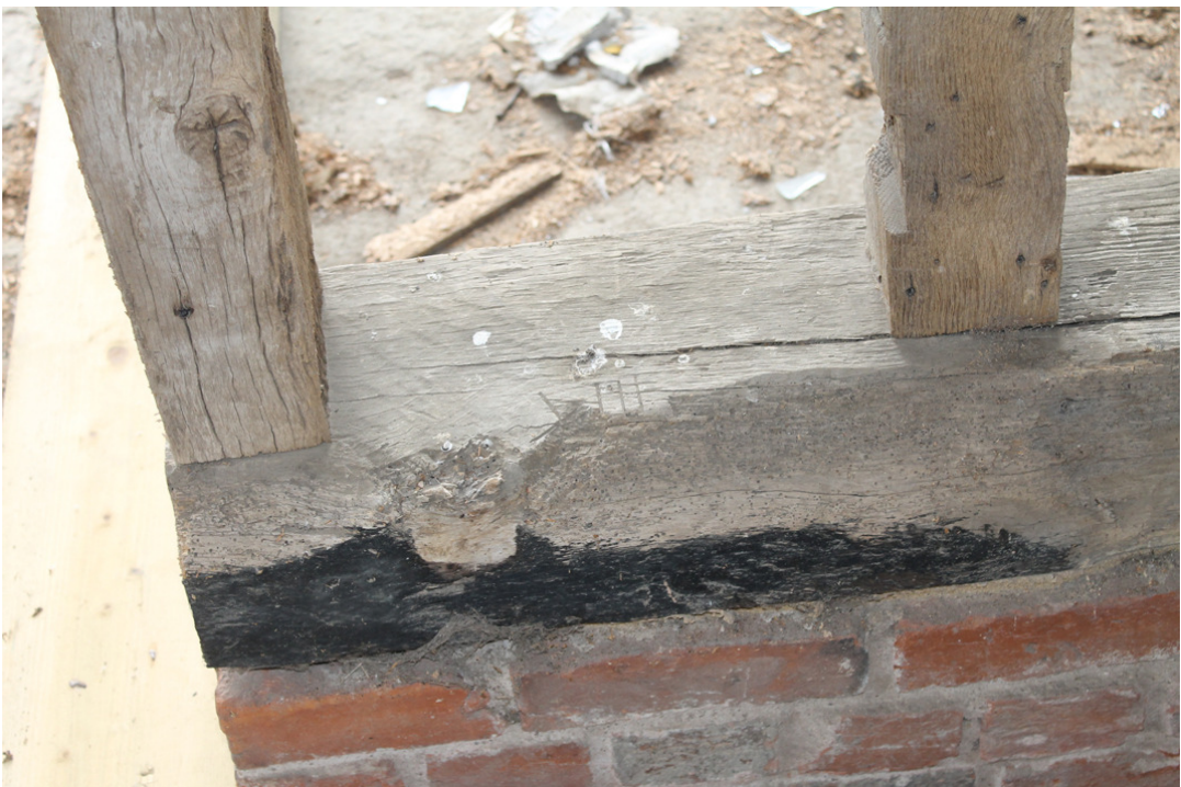
Photograph 18 Possible carpenter's mark out of context on a re-used timber forming part of the first floor addition in Bay 1. Photograph taken facing west.
