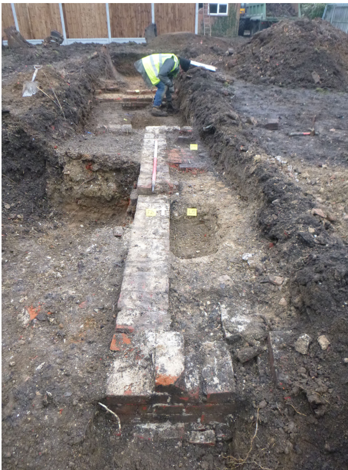
Photograph 1 Wall foundation F2, floor F5 and mortar base L5, looking NNW
