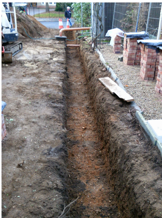
Photograph 1 Foundation trench for the brick wall, looking W
