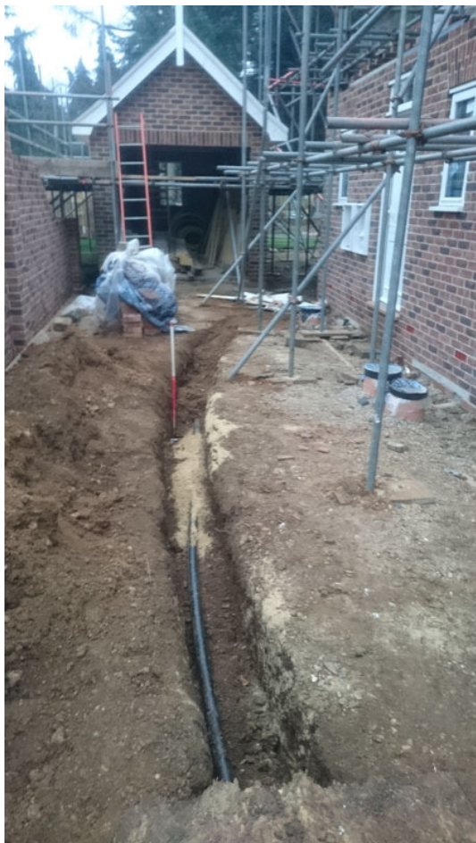
Photograph 2 Service trench, looking E
