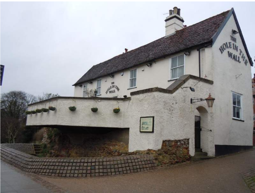
Plate 2 – Hole in the Wall Public House (Asset 3), the modern brick retaining wall around Balkerne Gate (Asset 2) is visible in the foreground
