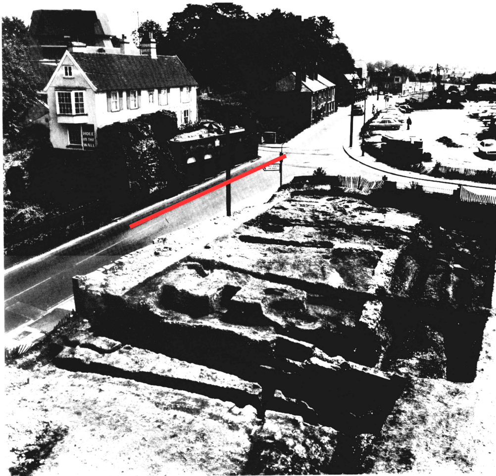
Photograph 3 Excavations at Balkerne Lane in the 1970s. The approximate location of piling to form the abutment wall for the eastern side of Balkerne Hill is shown in red, ground-level in front of that line reduced by approximately 6m for the new dual-carriageway (Colchester Archaeological Report 3, Figure 116).
