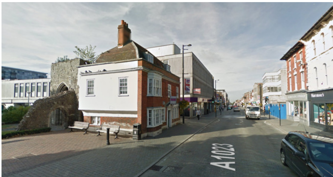
Photo 1: St Thomas' Chapel left, with a view SW down the High Street. The building right of the chapel is on the site of the Crown Inn (demolished 1927). The current site is behind the blue hoarding.
