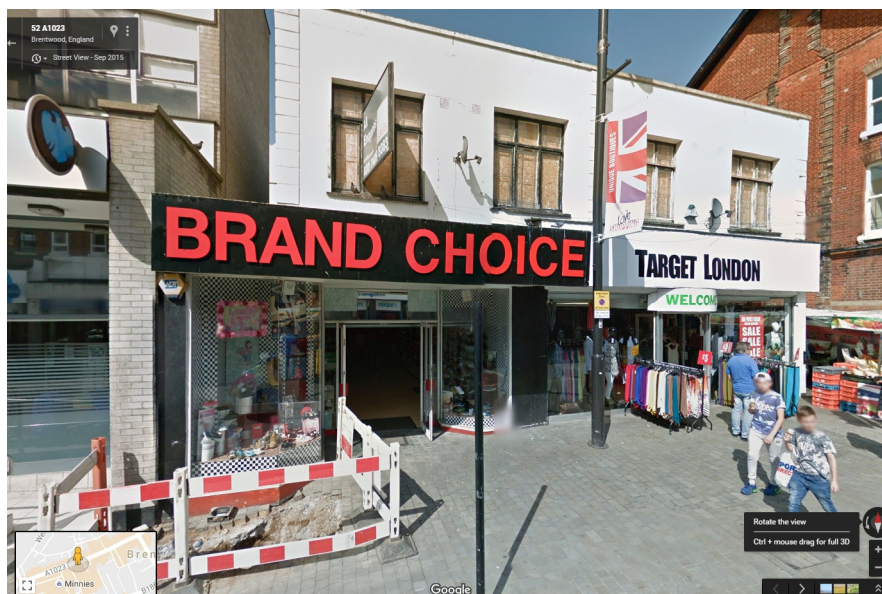
Photo 16: the site before the 2016 demolition
