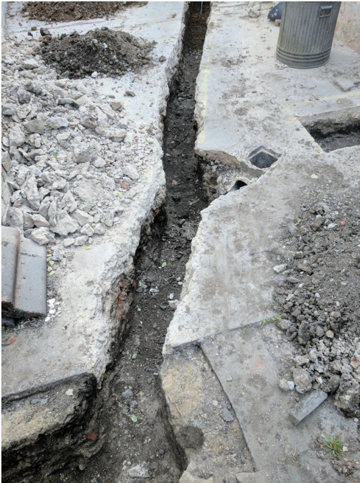
Photograph 2 Sewage trench, looking SSW
