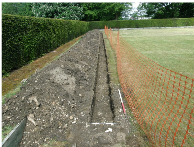
Photograph 2 T2 trench shot - looking north-west
