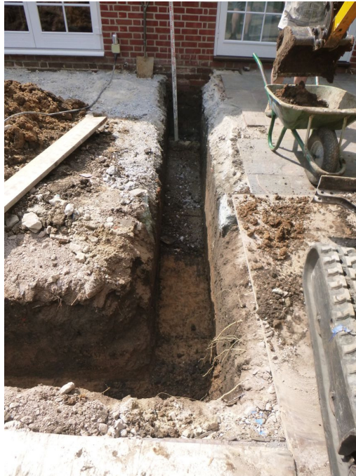
Photograph 1 North foundation - looking west
