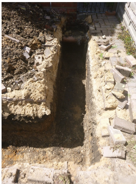
Photograph 1 Trench leg B - looking west
