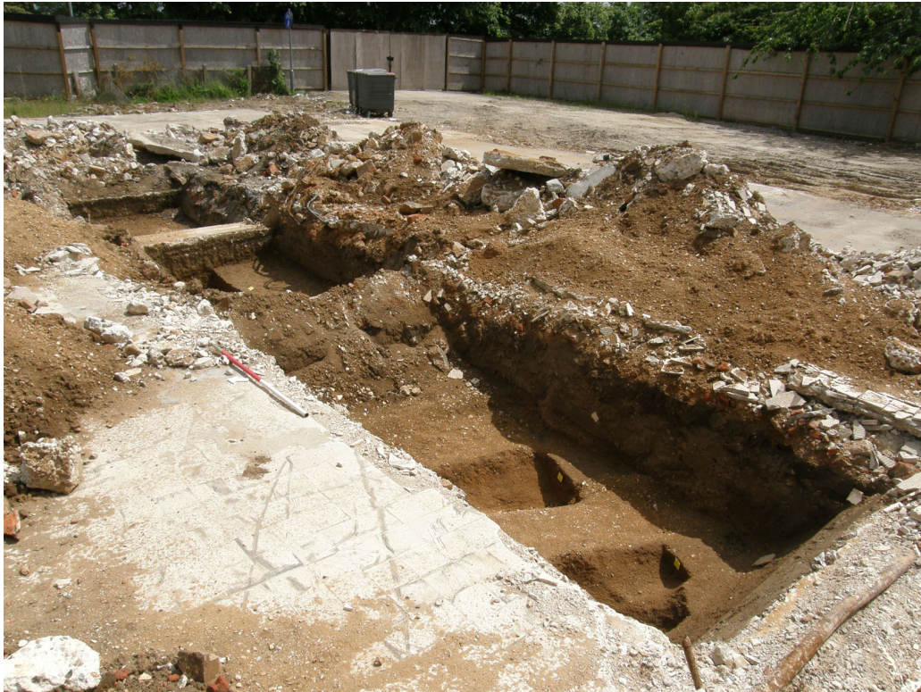
Photograph 4 Trench T17, looking E
