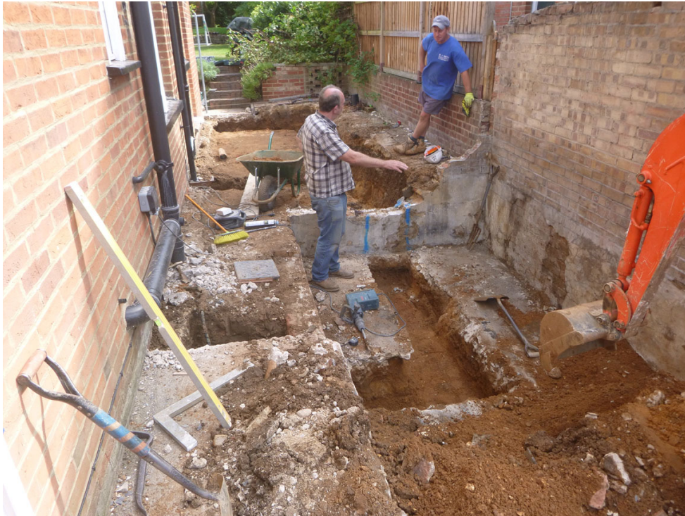
Photograph 2 Working shot showing trenched areas, looking southeast
