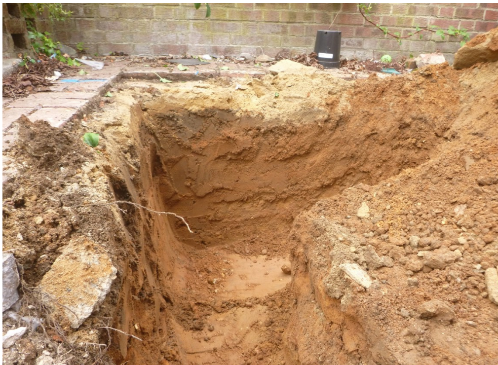
Photograph 1 Trench shot, looking west southwest
