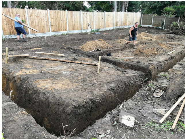
Photograph 1 Overview of finished trenches – looking southeast
