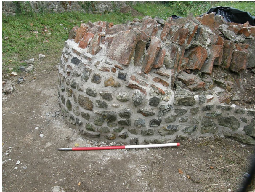
Photograph 7 Collapsed masonry after complete conservation. Photograph taken facing south-east.
