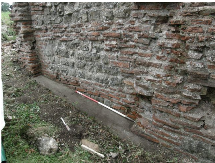
Photograph 8 Concrete drainage channel adjacent to the western side of Duncan's Gate. Photograph taken facing south-west.
