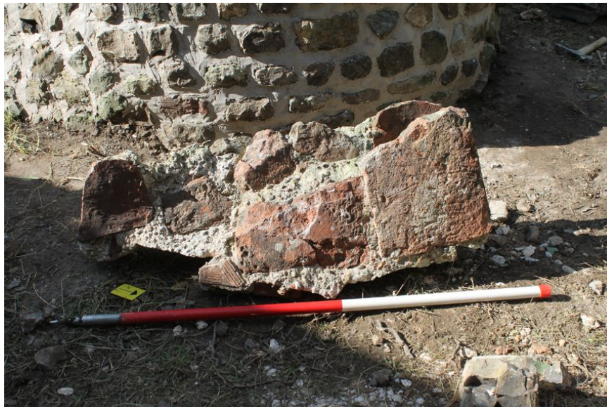
Photograph 3 Detail of tile courses that were successfully reattached together after falling.
