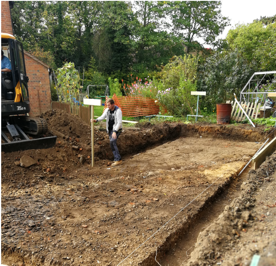
Photograph 1 Foundation trenches, looking N
