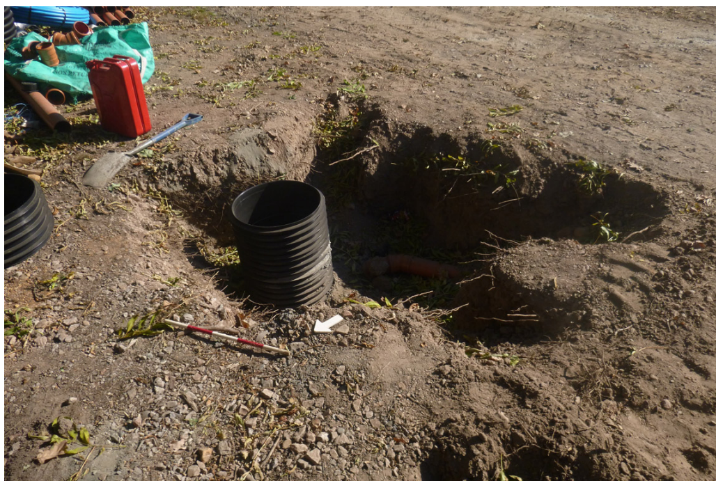
Photograph 2 Drainage hub, looking SE
