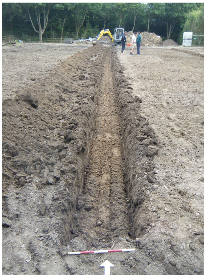
Photograph 1 Service trench, looking N
