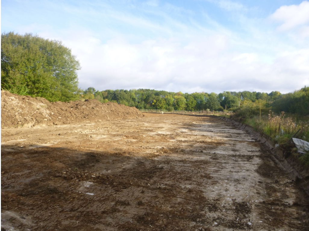
Photograph 1 Site shot showing reduction area
