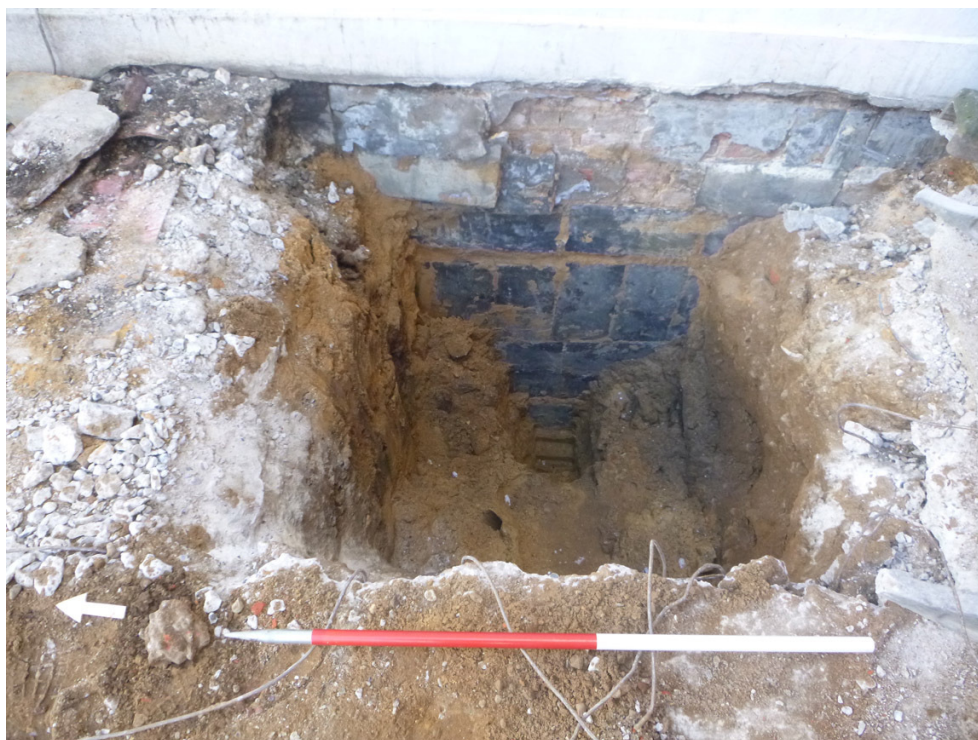
Photograph 2 Trial-hole 7, showing Town Hall foundations clad in slate, looking E
