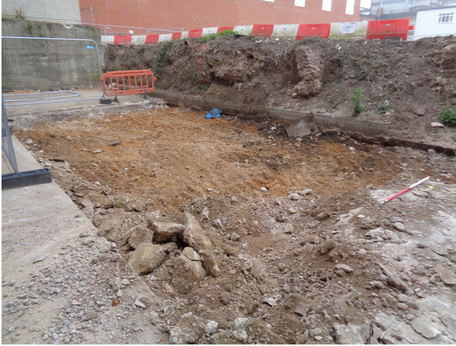
Photograph 3 Slab removal, looking NW
