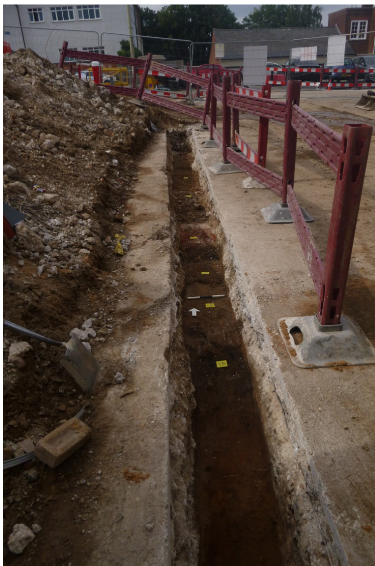
Photograph 8 UKPN service trench, looking N
