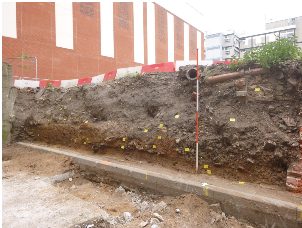
Photograph 5 Section (west end), looking NW
