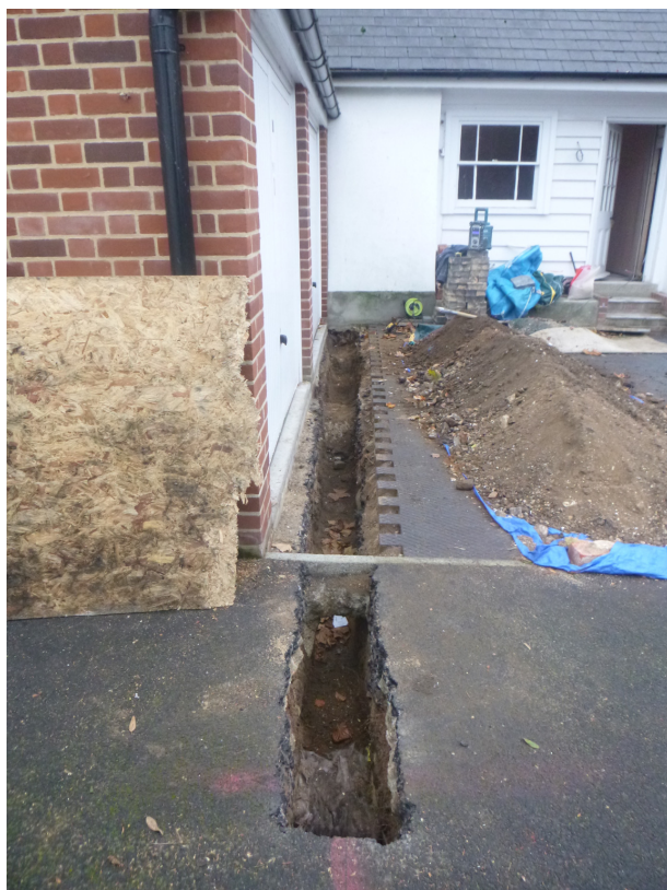
Photograph 1 Excavation of the service trench, view west
