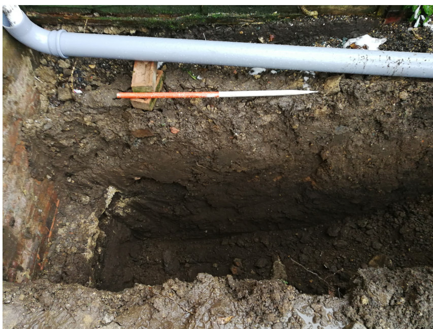
Photograph 4 Excavation of footings for new conservatory view west.
