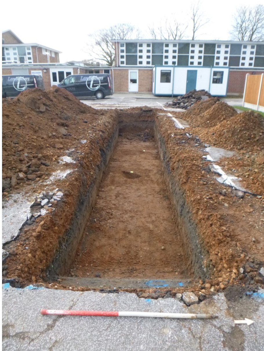
Photograph 2: T3 trench shot – looking west north-west
