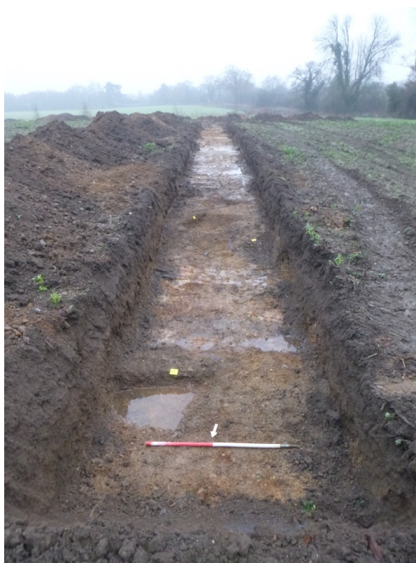
Photograph 1: T1 trench shot – looking south south-east
