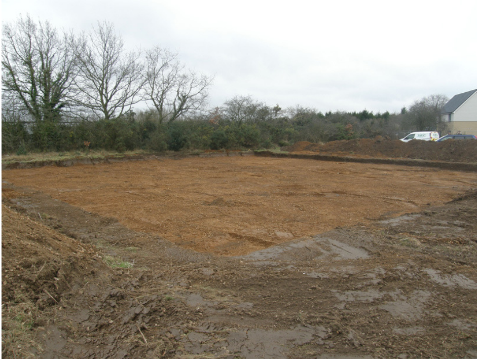
Photograph 3 Excavation Area C, looking S
