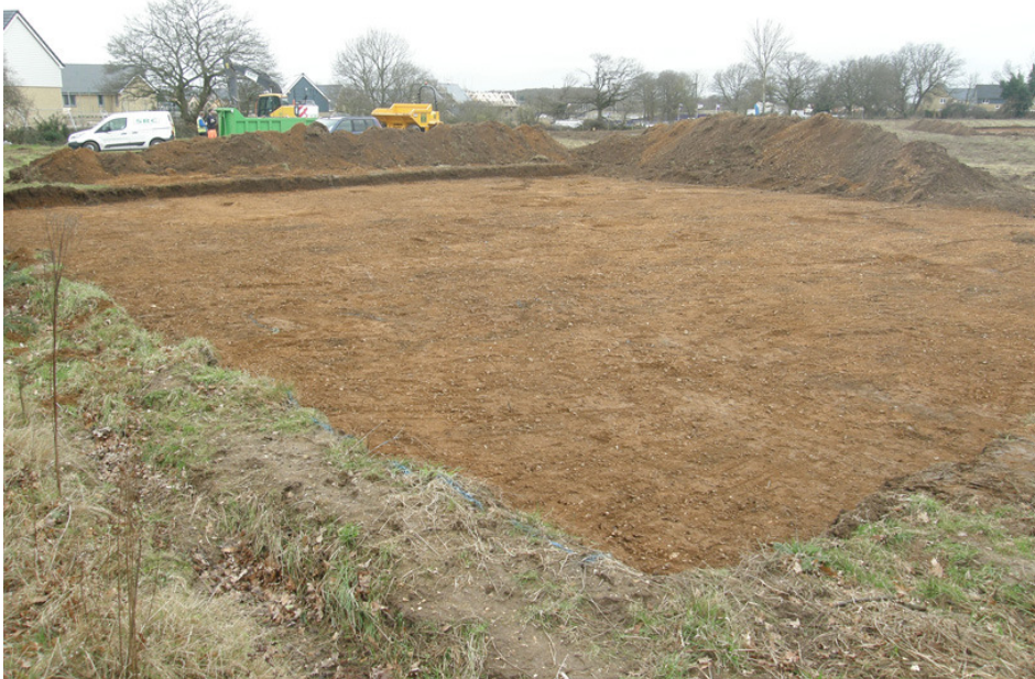
Photograph 2 Excavation Area B, looking S
