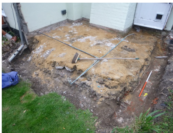
Photograph 2 Foundation trench oblique view – looking north north-west
