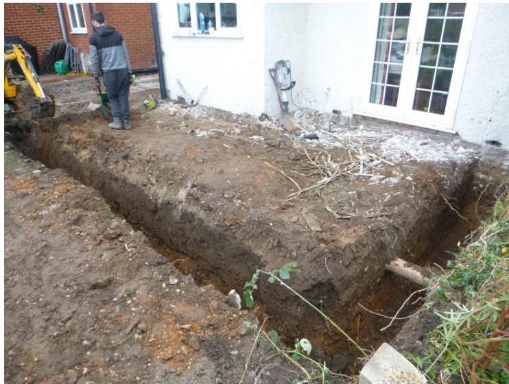
Photograph 1 Foundation trench, oblique view – looking west south-west
