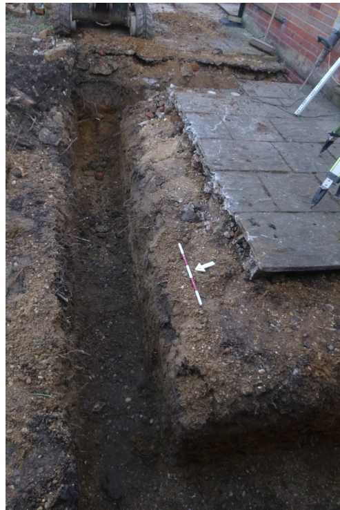
Photograph 1 Rear extension footing E-W branch – looking east south-east
