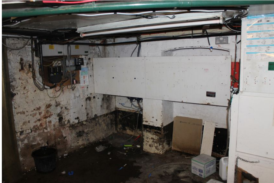
Photograph 14 Interior of cellar, showing brick arch supporting chimney-stack on upper floors. Photograph taken facing east.
