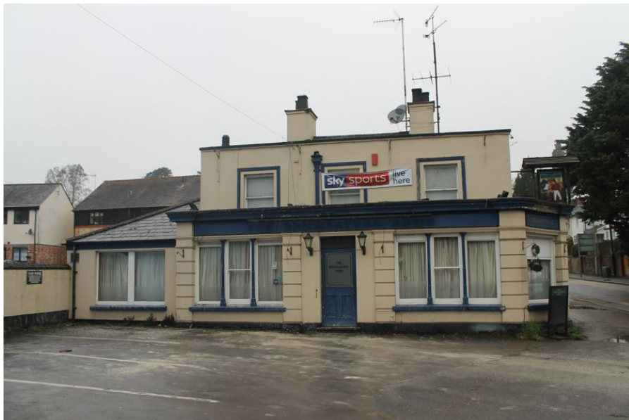
Photograph 7 South-east elevation of Bricklayers Arms. Photograph taken facing north-west.
