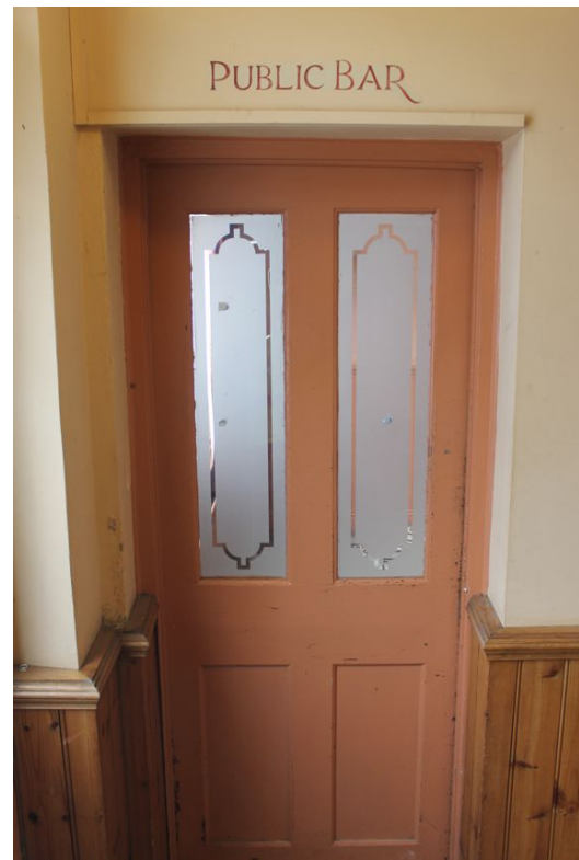
Photograph 17 Four-panel door leading to the southern bar from the foyer (the decal labelling this as the "Public Bar" is a modern addition, as this bar would almost certainly have been the lounge bar). Photograph taken facing south-west.
