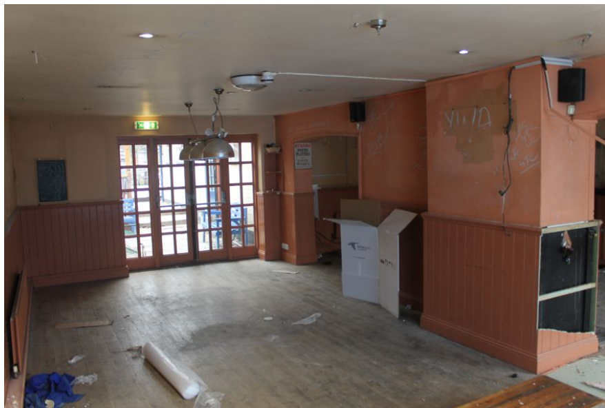
Photograph 15 Interior of extension B, showing dado-rail and blocked fireplace. Photograph taken facing north-west.
