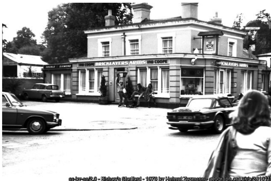
Photograph 4 Bricklayers Arms in 1973. Inserted windows in place of original double doorway on the pub, and on extension B, both visible. Pub owned by Ind Coope. From www.geograph.org.uk .
