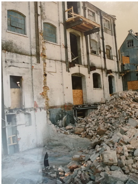
Photograph 4 Showing rubble during mill conversion, looking southeast
