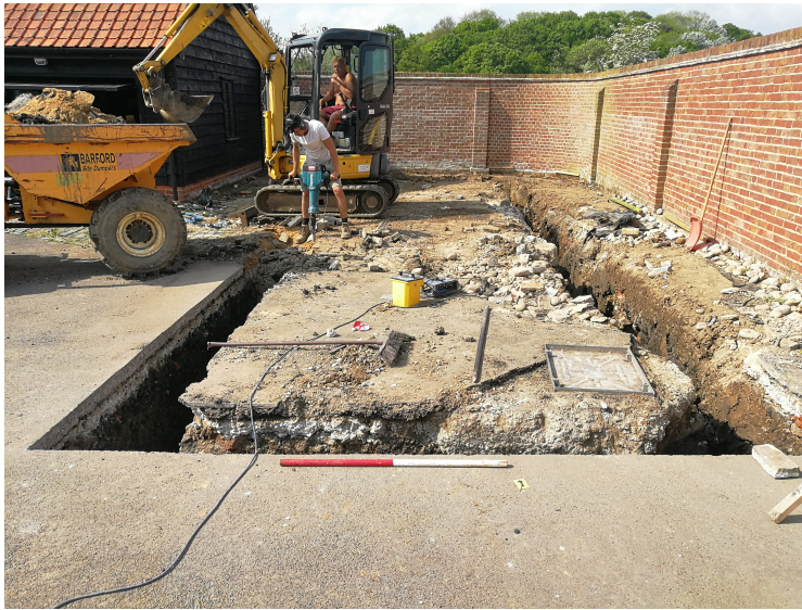
Photograph 1 Foundation trench, looking north northwest
