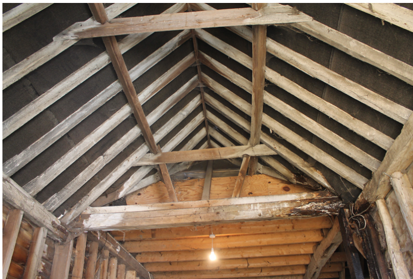
Photograph 14 Tie-beam between bay 3 and midstrey. Photograph taken facing west.
