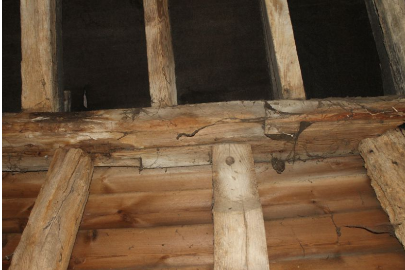
Photograph 20 Scarf joint on western wall-plate of bay 2. Photograph taken facing west.
