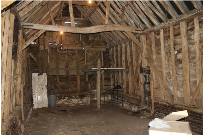
Photograph 8 Interior of barn, showing bays 1 and 2. Photograph taken facing north-east.
