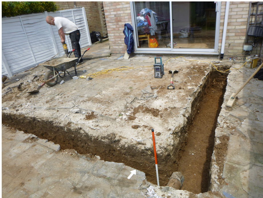
Photograph 1 The site of the extension – looking north-west
