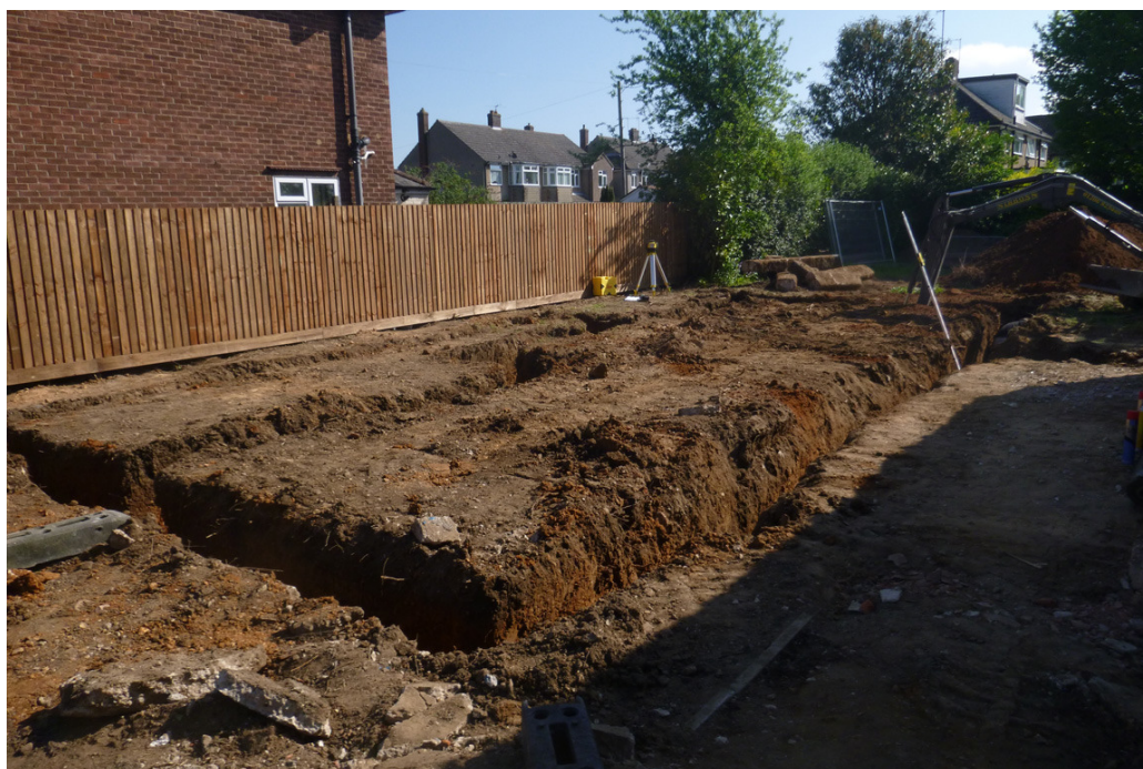
Photograph 1 Foundation trenches, looking NE
