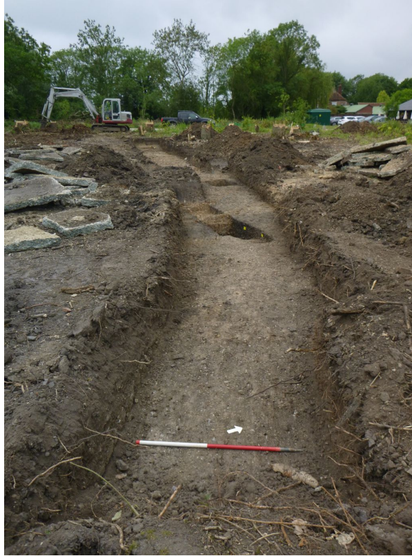
Photograph 7 Long shot of T4, showing gravelly natural L3 and F10, F11 and F12. Photograph taken facing north-west.
