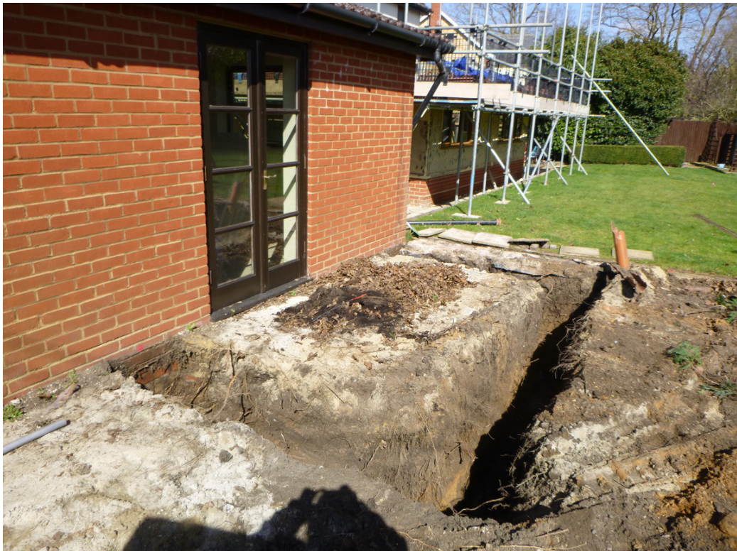
Photograph 1 Foundation trenches, looking northwest
