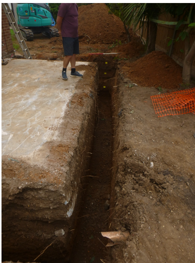
Photograph 1 N-S branch of foundation trenching, looking north
