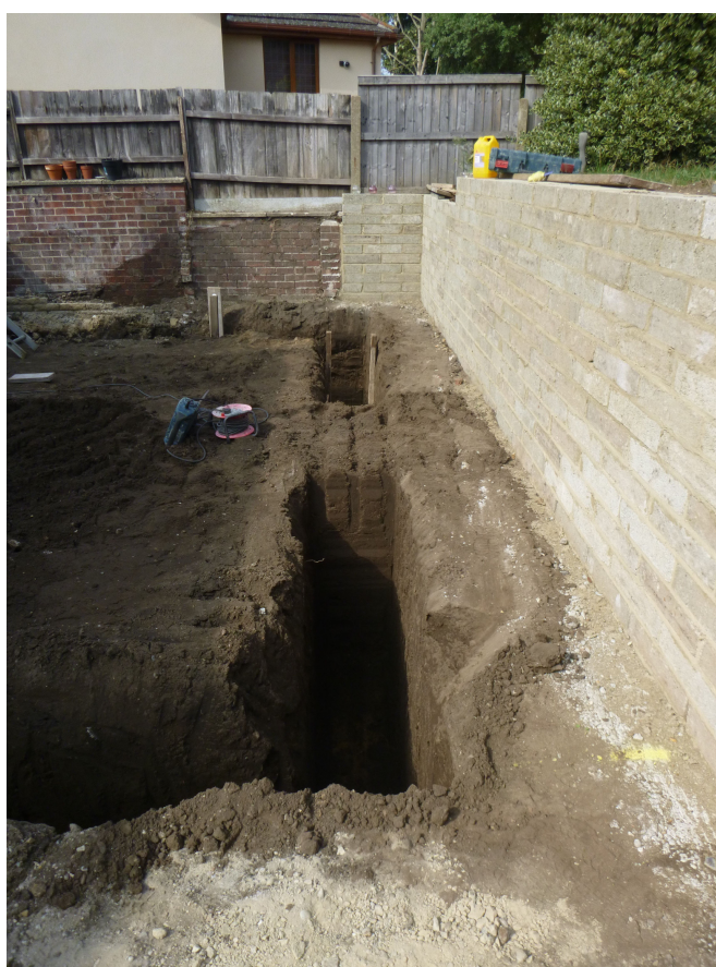
Photograph 1 N-S branch of foundation trenching – looking north
