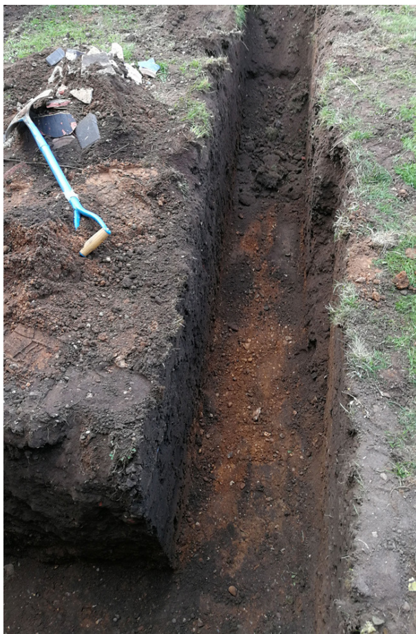
Photograph 1 Foundation trench, looking southwest
