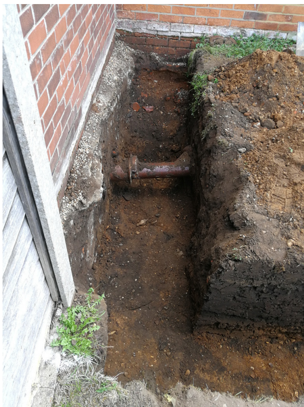
Photograph 2 Foundation trench, looking southeast
