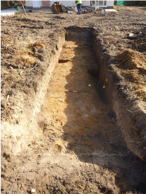
Photograph 1 Trench T2, looking east
