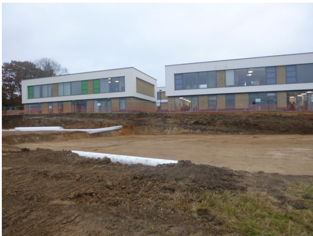
Photograph 2 Level reduction of Block F, looking NE
