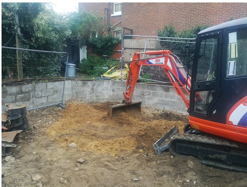
Photograph 1 Working shot, looking southeast
