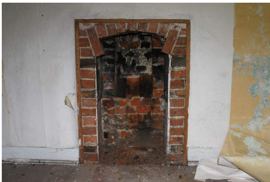
Photograph 18 Original brick fireplace in north-east room on the first-floor of the Rising Sun. Photograph taken facing north-east.
