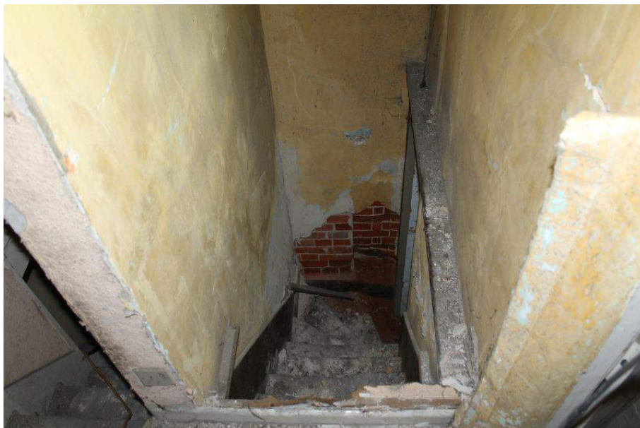
Photograph 30 Southern staircase, view from the first-floor. Note top step is boarded over. Timber to right of frame would have supported boards covering whole staircase. Also visible at bottom of staircase is exposed brickwork with joint and queen closers. Photograph taken facing north-east.
