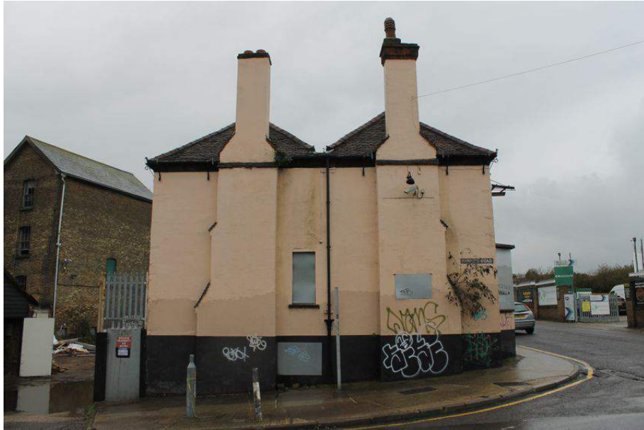
Photograph 6 North-east elevation of the Rising Sun (Structure 1). Photograph taken facing south-west.
