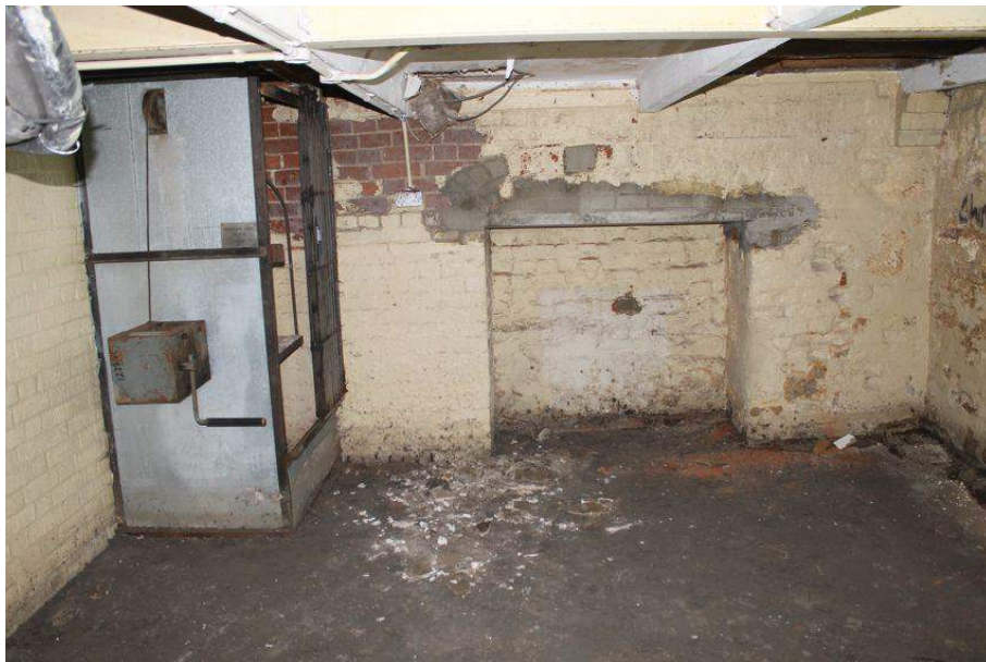
Photograph 8 Basement of Rising Sun (Structure 1). Showing north-west fireplace and inserted dumb waiter. Photograph taken facing south-west.
