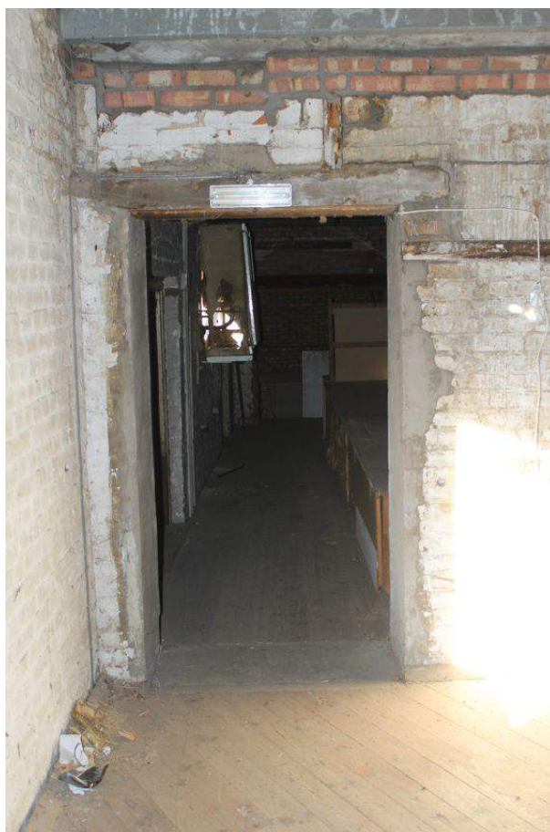
Photograph 80 Entrance into second-floor of Structure 7, showing differing floor-levels. Photograph taken facing north.
