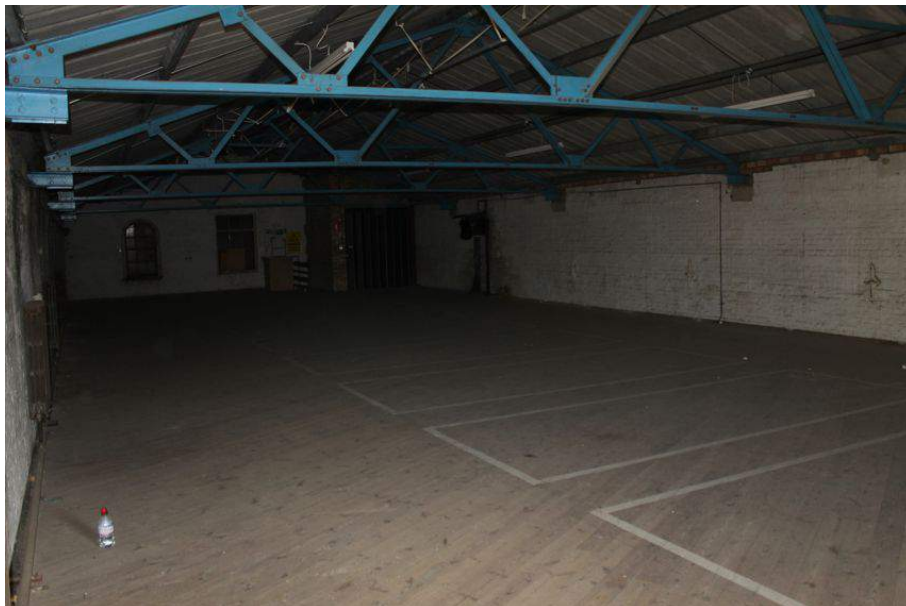
Photograph 90 Second-floor of Structure 8. Photograph taken facing south-east.
