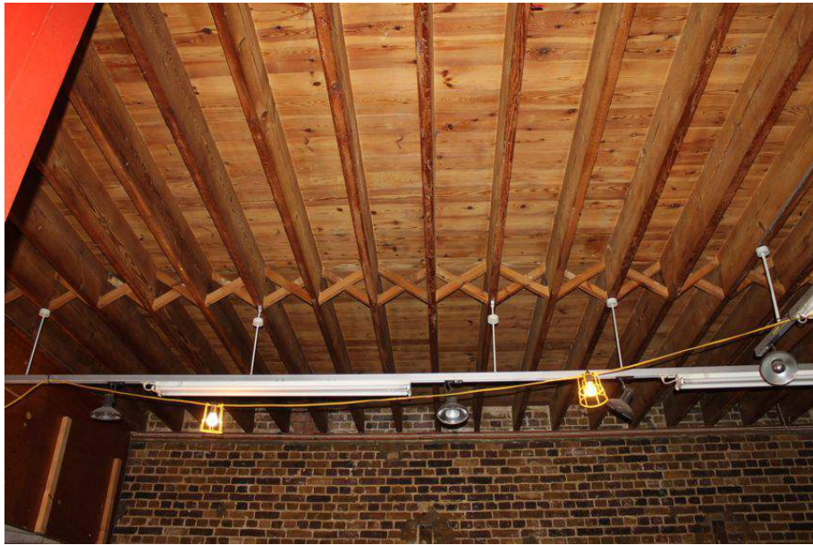
Photograph 76 Herringbone strutting supporting first-floor of Structure 7. Photograph taken facing south.
