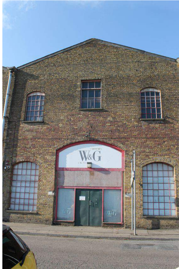
Photograph 67 East elevation of Structure 7. Photograph taken facing west.
