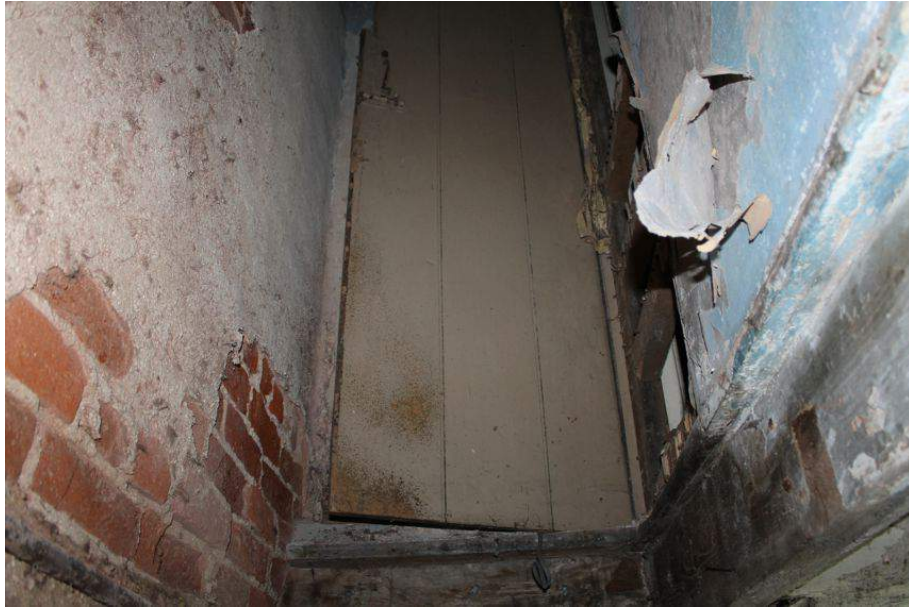
Photograph 25 View of original door on ground-floor from location of removed stairway in basement of Structure 2. Photograph taken facing south-west.
