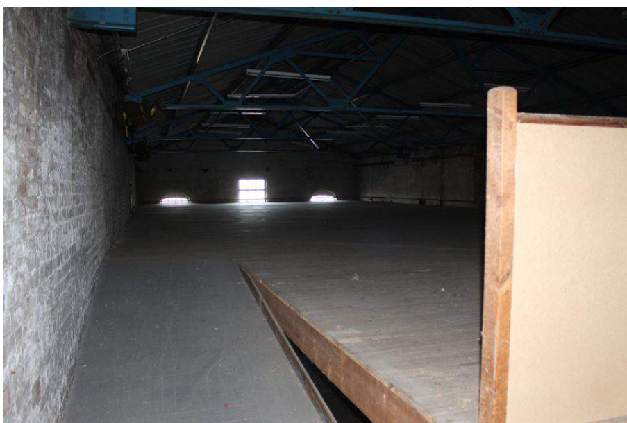
Photograph 81 Second-floor of Structure 7. Ramp visible in foreground. Photograph taken facing east.
