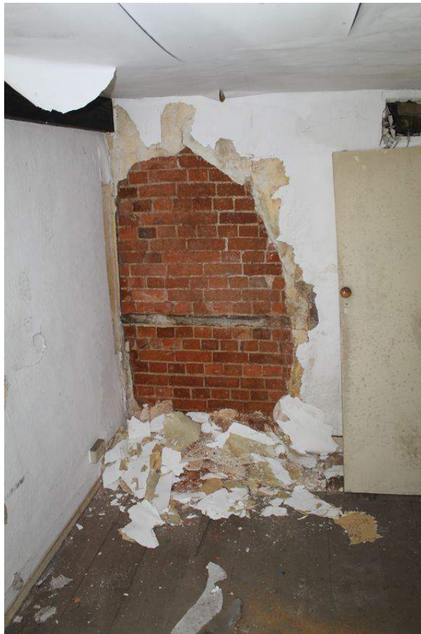
Photograph 17 Exposed English-bond brickwork on first-floor of Rising Sun. Photograph taken facing north-east.
