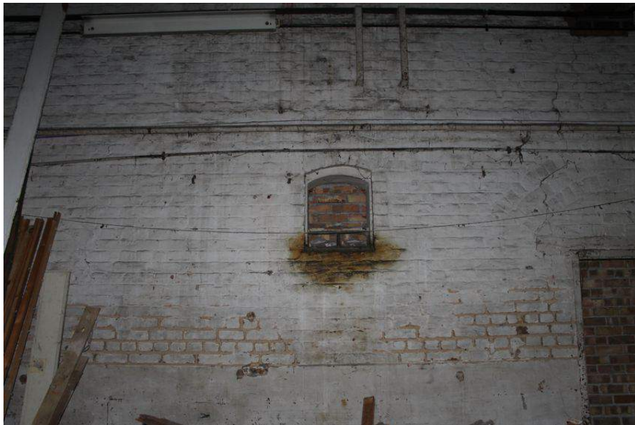
Photograph 63 Possible metal-framed ?gas-light holder in recess in south ground-floor wall of Structure 6. Photograph taken facing south.
