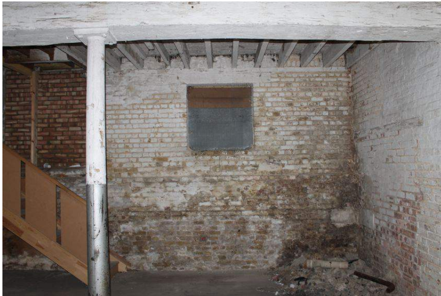
Photograph 87 Western wall in ground-floor of Structure 8, showing blocked western doorway, and its height above floor-level, to left of frame. Also visible is a blocked window and another blocked opening in the northern wall to the right. Photograph taken facing west.
