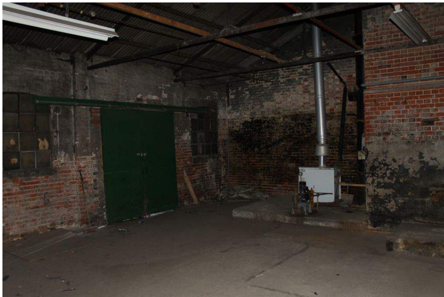
Photograph 93 Interior of Structure 9. Photograph taken facing south-east.
