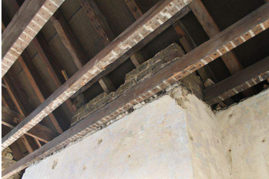
Photograph 52 Top of chimney-stack in Structure 5, having been removed to below the rafters. Note the modern rafters above it. Photograph taken facing north-west.
