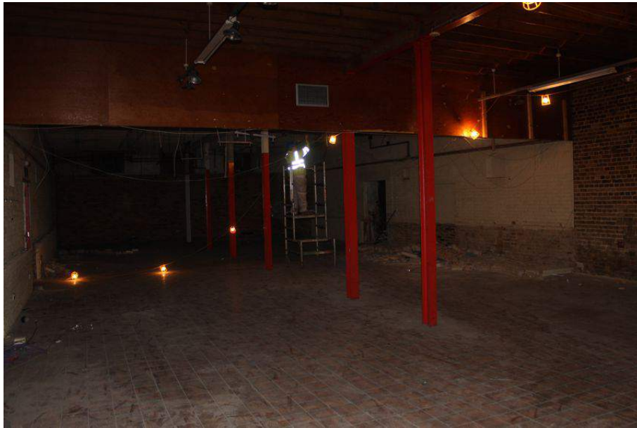
Photograph 71 Ground-floor of Structure 7. Photograph taken facing north-west.
