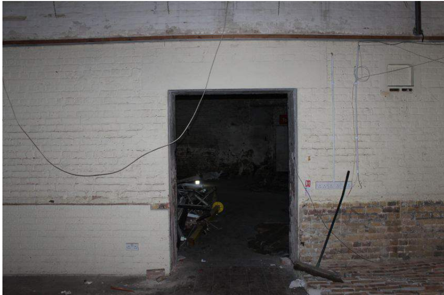
Photograph 61 Inserted entrance with a concrete lintel between Structures 6 and 7 on the ground-floor. Photograph taken facing north.
