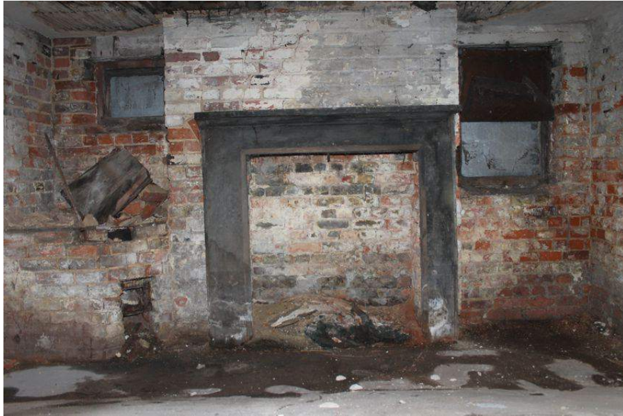
Photograph 42 Fireplace in eastern room of basement in Structure 5. Note carved wooden surround. Water heater visible to left. Photograph taken facing north.
