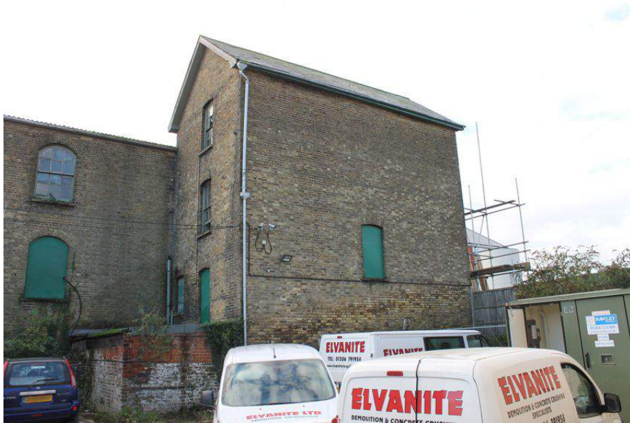
Photograph 38 Northern elevation of four-storey house (Structure 5). Photograph taken facing south-west.
