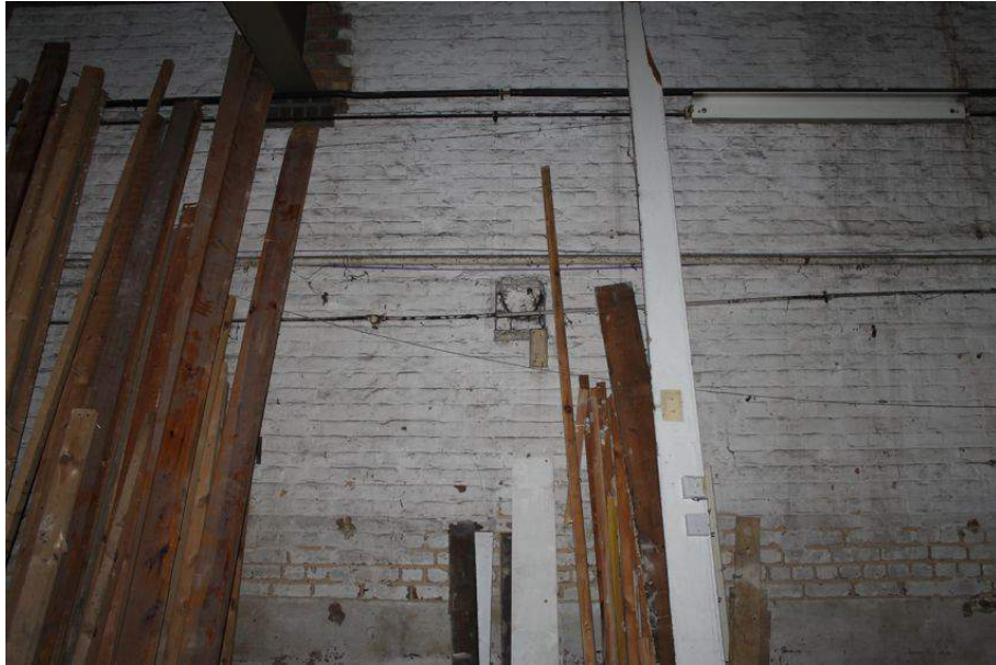
Photograph 60 Recess in southern ground-floor wall of Structure 6, possibly to support a binding-beam for the original floor. Photograph taken facing south.
