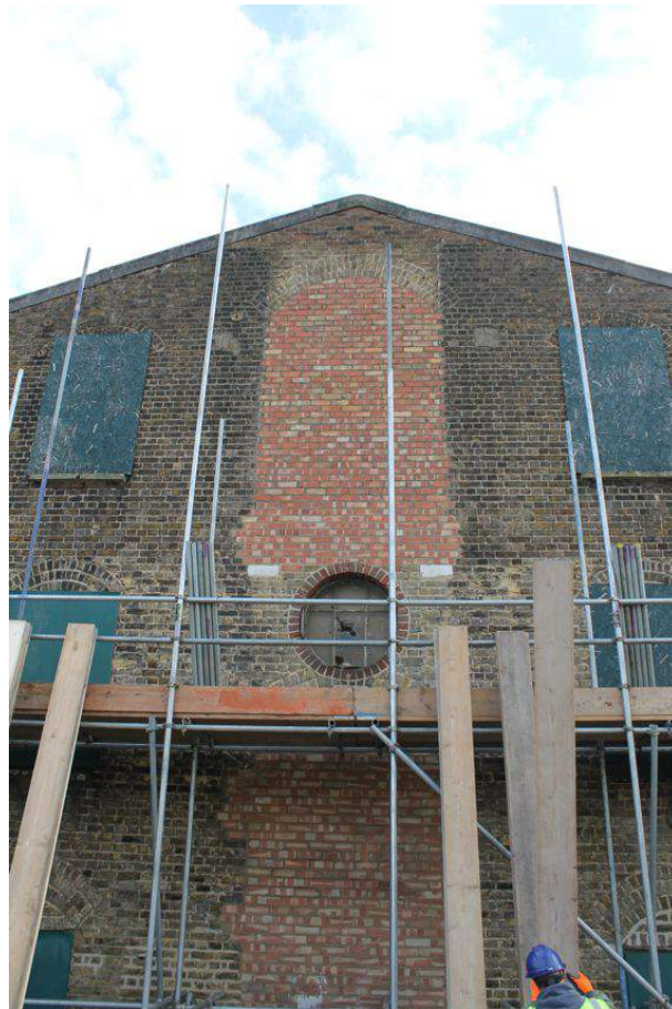
Photograph 84 Western elevation of Structure 8. Modern brickwork shows location of removed lift and entrance shown in Photograph 4. Photograph taken facing east.
