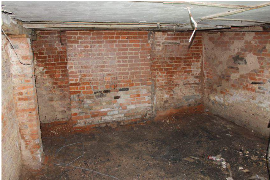
Photograph 26 Northern room of Structure 2's basement, showing west wall of Rising Sun. Note the central structural wall of the house extension (to right) is not bonded to the pub's walls. Photograph taken facing east.
