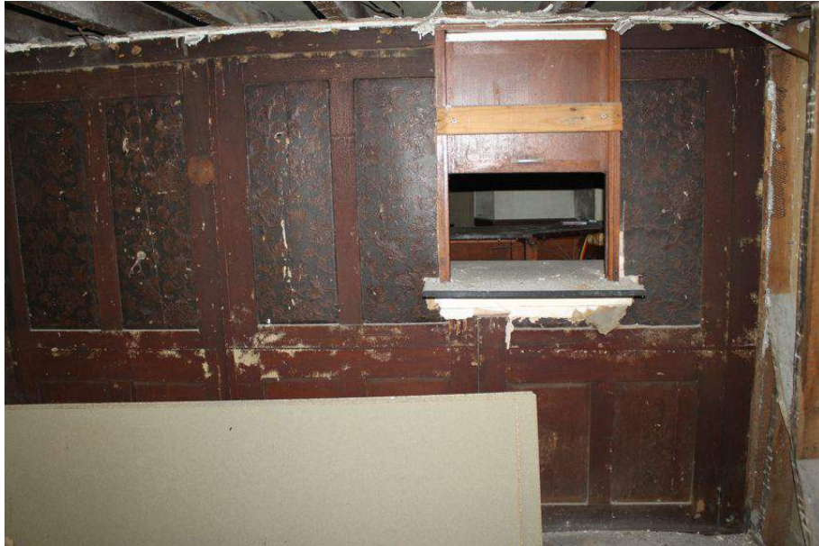
Photograph 14 Decorated wooden panels and inserted serving hatch in south-west room on ground-floor of Rising Sun. Photograph taken facing north-west.
