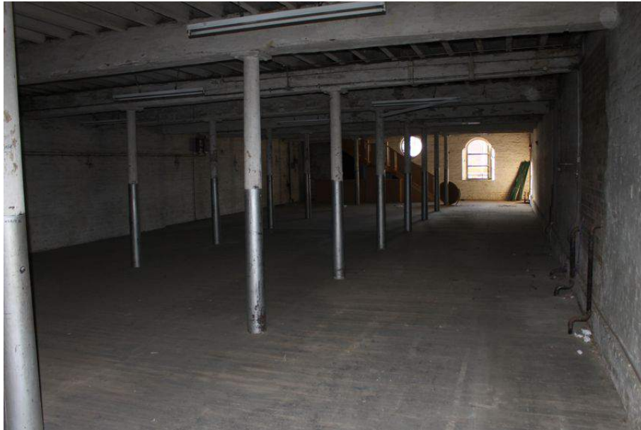
Photograph 89 First-floor of Structure 8. Photograph taken facing south-west.
