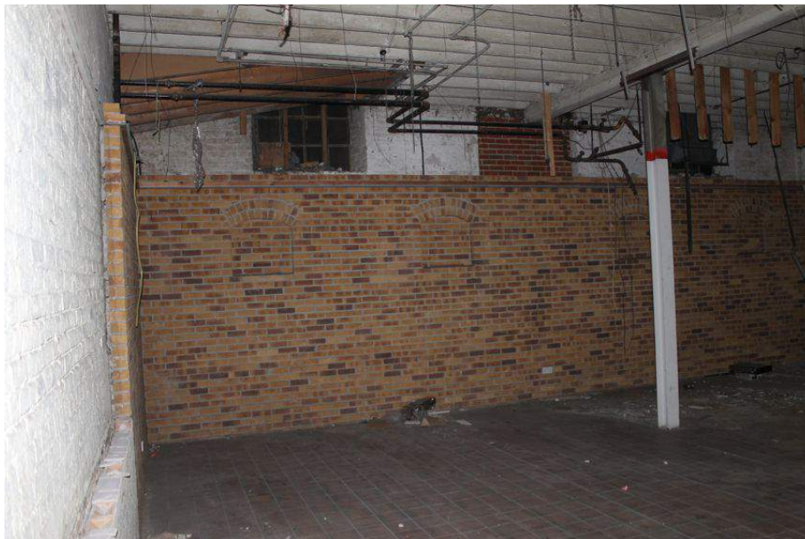
Photograph 72 Modern skin of bricks over original brickwork in western end of Structure 7. Entrance and windows on western elevation also visible. Photograph taken facing north-west.
