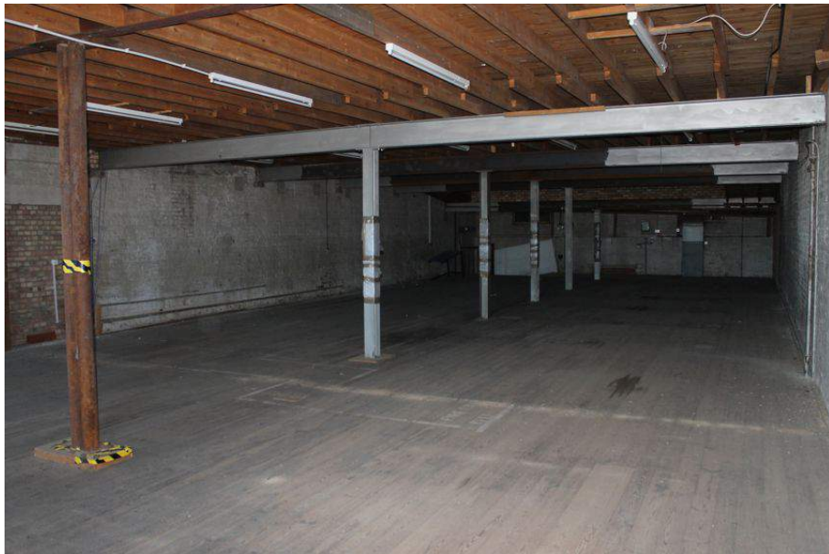
Photograph 77 First-floor of Structure 7. Photograph taken facing south-west.
