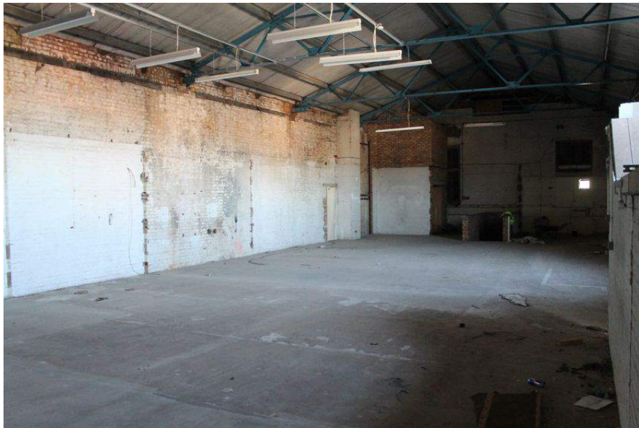
Photograph 65 First-floor of Structure 6. Photograph taken facing south-west.
