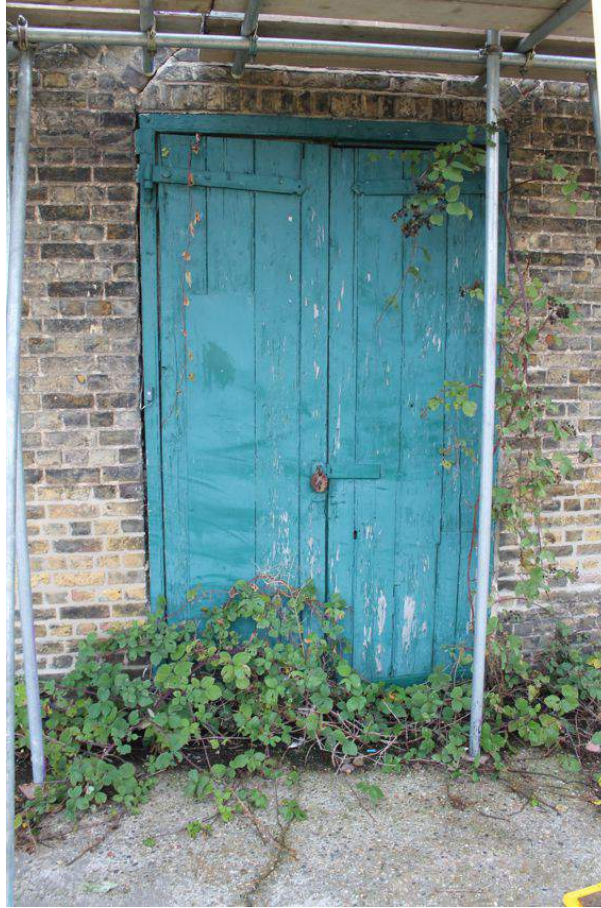
Photograph 69 Vertical-planked door on western elevation of Structure 7 (blocked from the inside). Photograph taken facing east.
