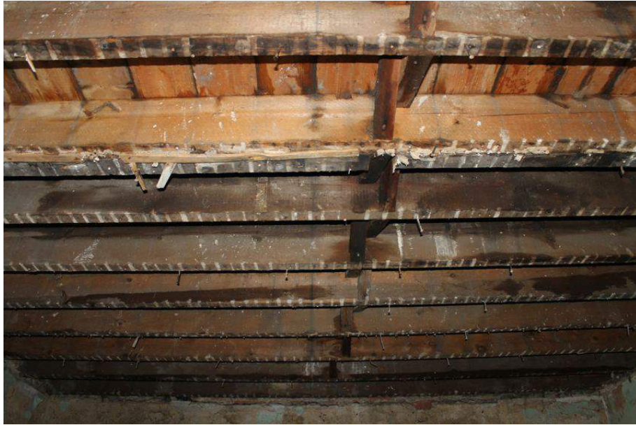
Photograph 48 Underside of second-floor in Structure 5, showing supporting herringbone-strutting. Photograph taken facing north.
