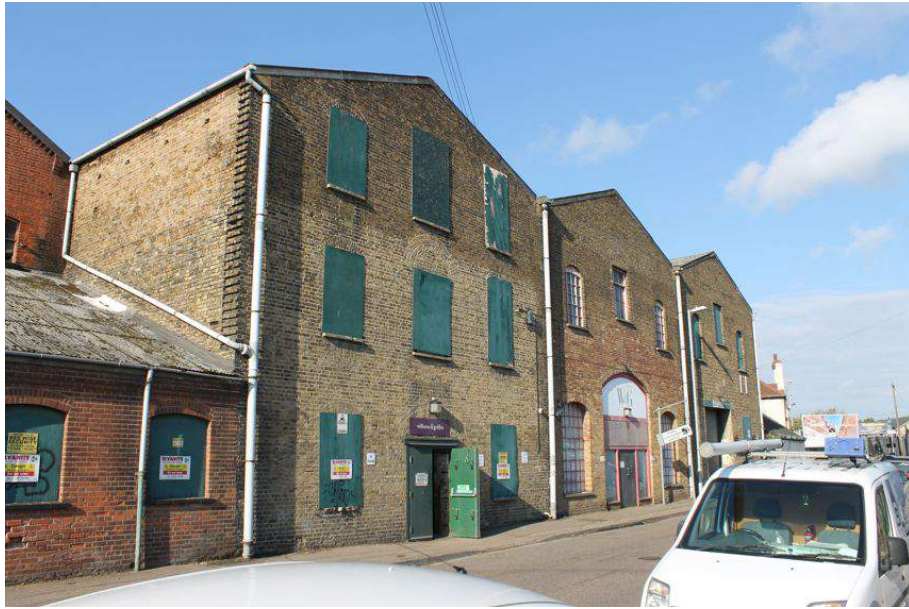
Photograph 66 East elevation of warehouse range. Structure 8 to left, Structure 6 to right. Photograph taken facing north-west.
