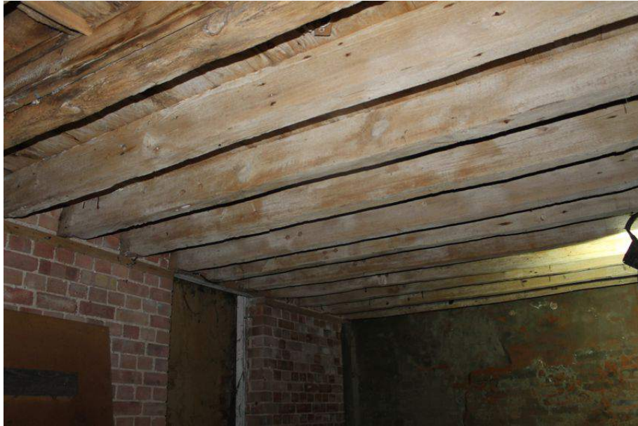
Photograph 27 Joists supporting ground-floor, view from southern room of basement in Structure 2. Photograph taken facing south.
