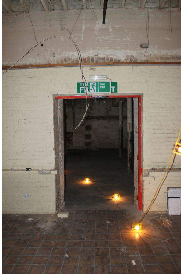
Photograph 73 Original entrance on ground-floor between Structures 7 and 8. Archway above. Photograph taken facing south.
