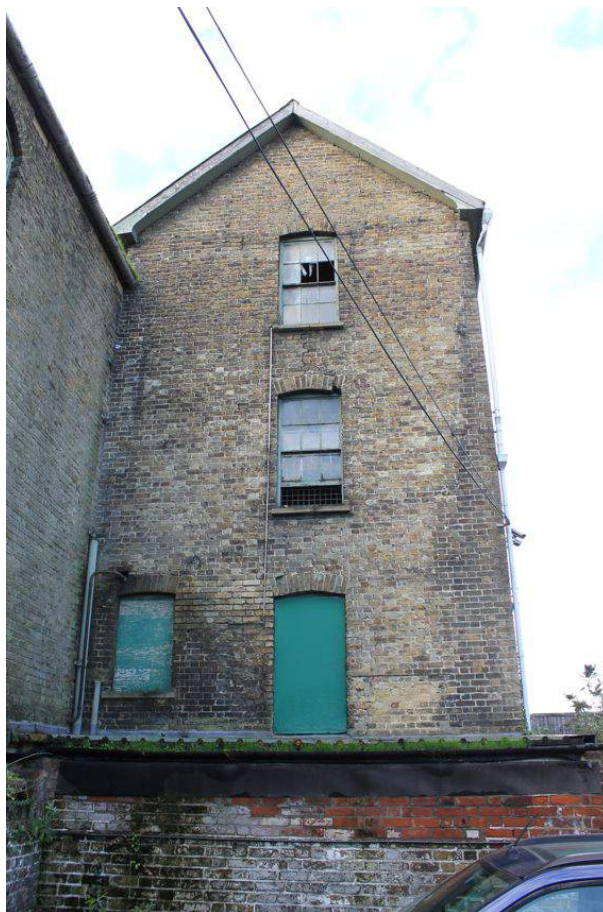
Photograph 39 Eastern elevation of Structure 5. Photograph taken facing west.
