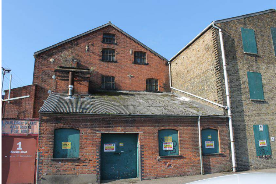
Photograph 92 East elevation of Structure 9. Photograph taken facing west.
