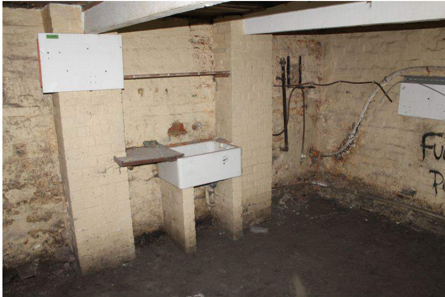
Photograph 10 Basement of the Rising Sun, showing inserted brick plinths supporting modern beams in north-east room. Photograph taken facing south-east.
