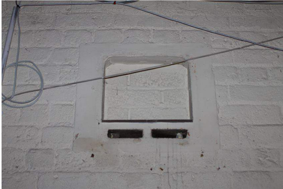
Photograph 74 Possible ?gas-light holder in northern brickwork on ground-floor of Structure 7. Photograph taken facing north.
