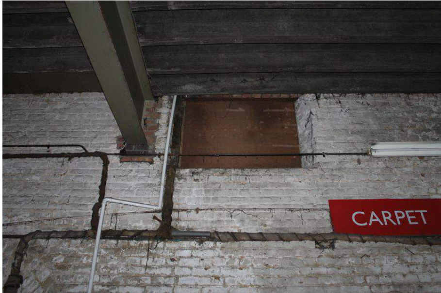
Photograph 64 Metal-beam supporting inserted first-floor of Structure 6, adjacent to a bisected window opening. Photograph taken facing north.
