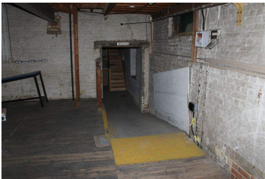
Photograph 79 Entrance between Structures 7 and 8 on first-floor. Photograph taken facing south-west.
