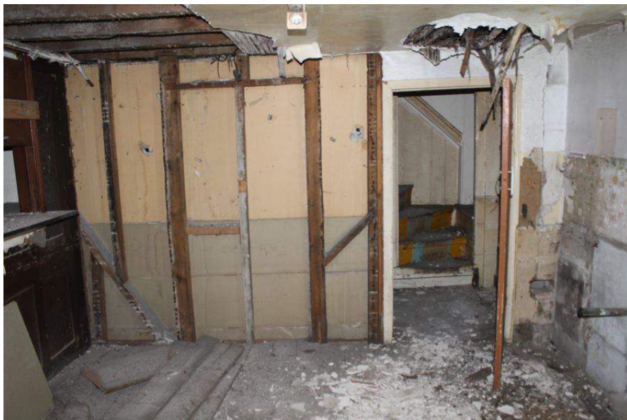
Photograph 15 Eastern wall of south-west room on ground-floor of Rising Sun. Blocked doorway visible to left of frame, inserted doorway visible to right. Photograph taken facing north-east.
