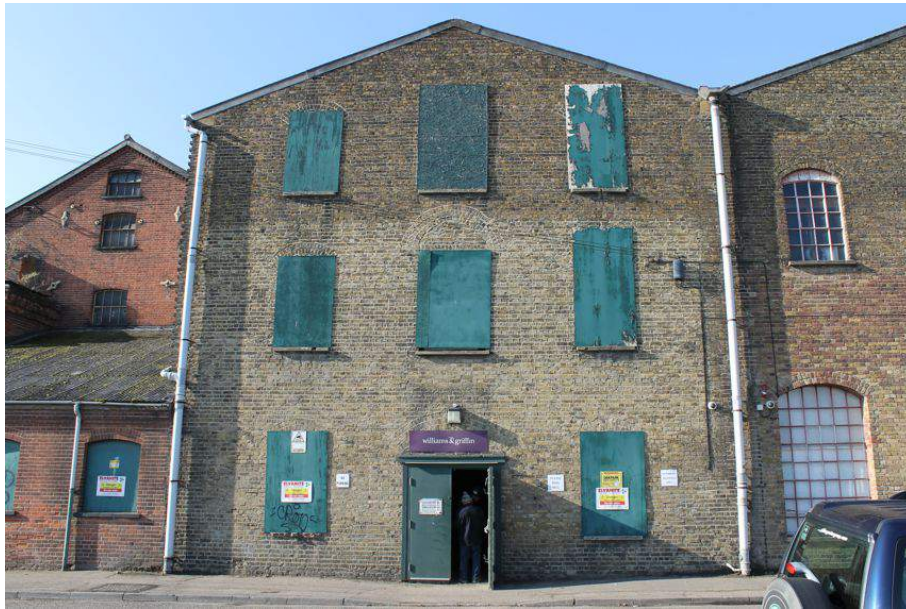
Photograph 82 East elevation of Structure 8. Photograph taken facing west.
