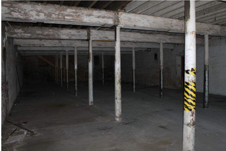
Photograph 85 Ground-floor of Structure 8. Photograph taken facing north-west.
