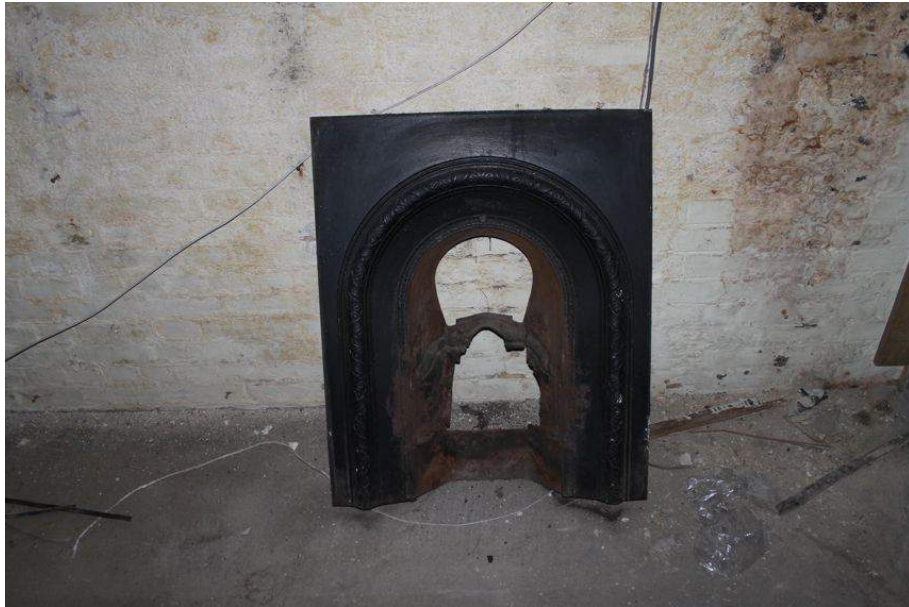
Photograph 50 Metal register grate taken from fireplace on first-floor of Structure 5.
