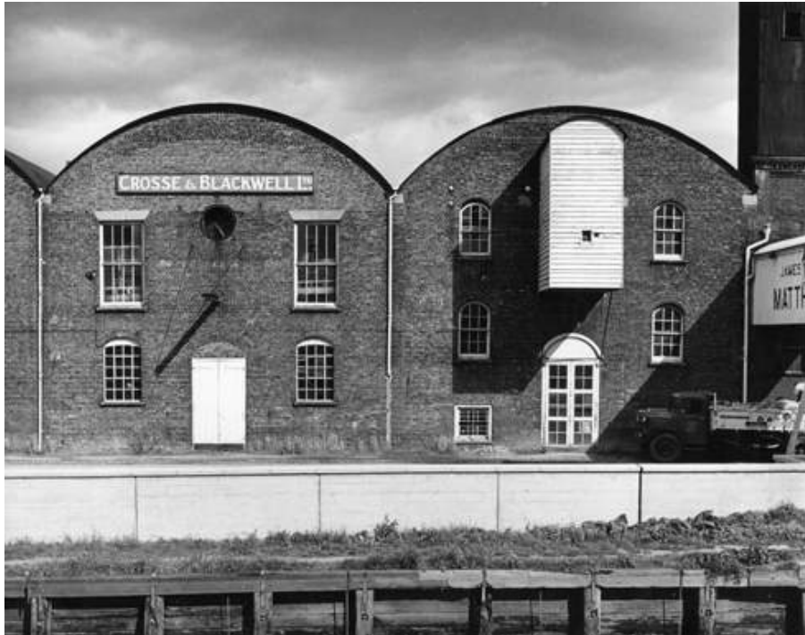
Photograph 4 West elevation of warehouses in 1956 (Structures 7 and 8), showing original barrel roofs. Shows warehouses were occupied by Crosse and Blackwell Ltd. Also visible is the lift on the frontage of Structure 8. The large chimney in the top right, rising from the adjacent warehouse, is much taller than it is today.
