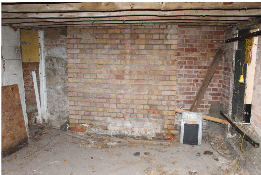
Photograph 21 Rebuilt chimney-stack of Rising Sun, visible in basement of Structure 2. Photograph taken facing east.
