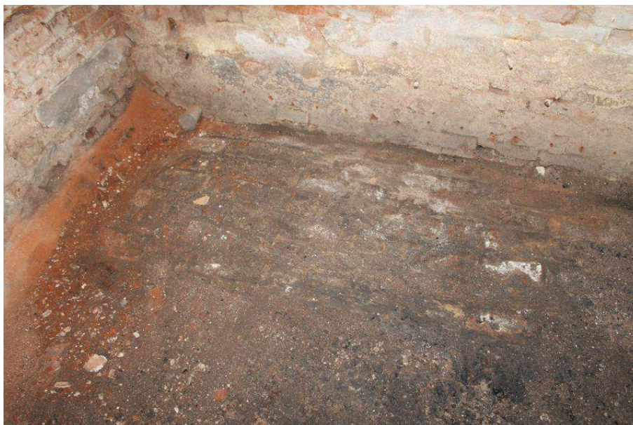
Photograph 22 Surviving section of pavior-brick floor in northern room of house extension's (Structure 2's) basement. Photograph taken facing south-east.
