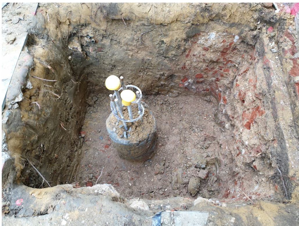
Photograph 5 Groundbeam 1, showing F4 on right-hand side, looking northeast
