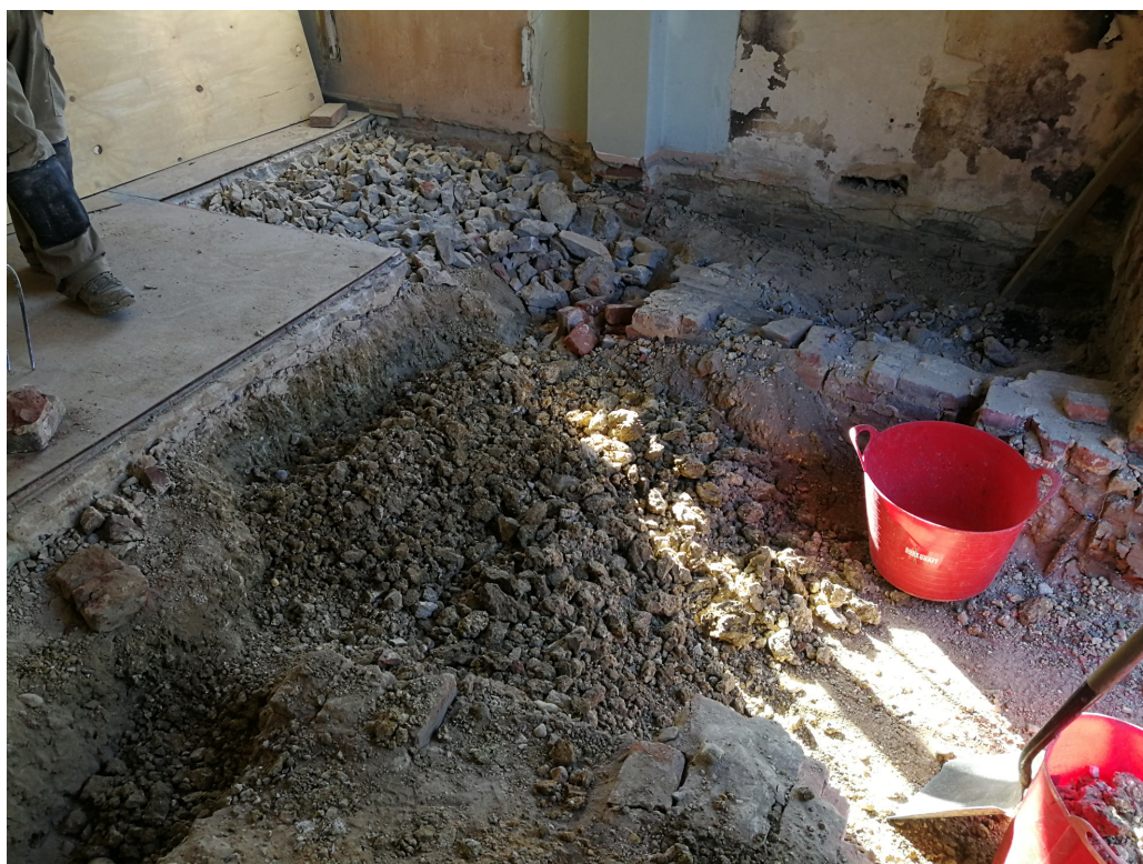
Photograph 3 Ground reduction within the extension, looking southwest
