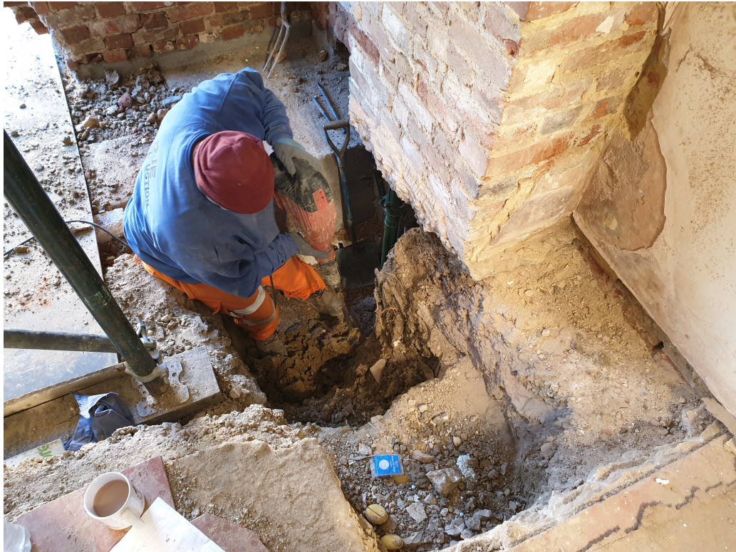
Photograph 7 Excavation of groundbeam slots to underpin the chimney, looking north
