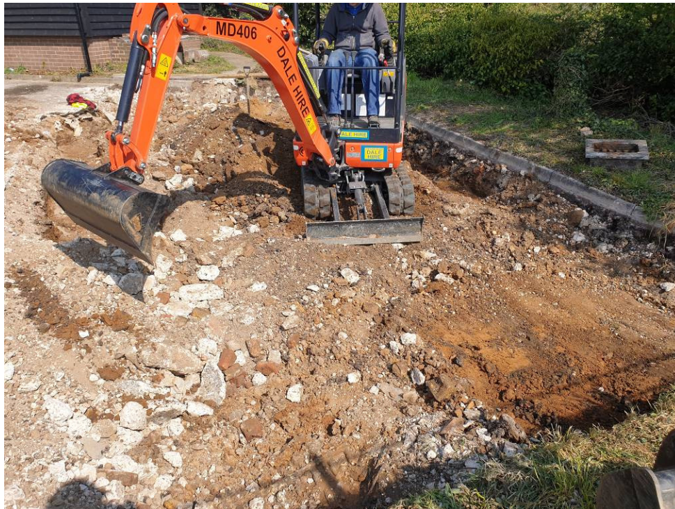
Photograph 1 Working shot, looking northeast
