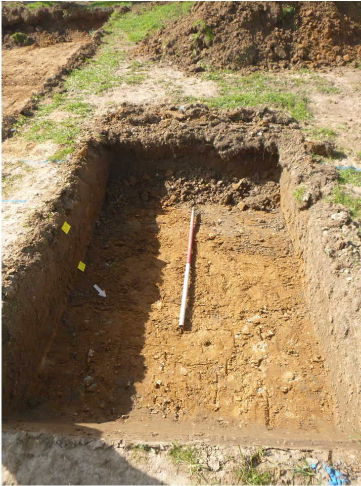
Photograph 2 Site shot of the excavation area for electricity sub-station, looking southwest
