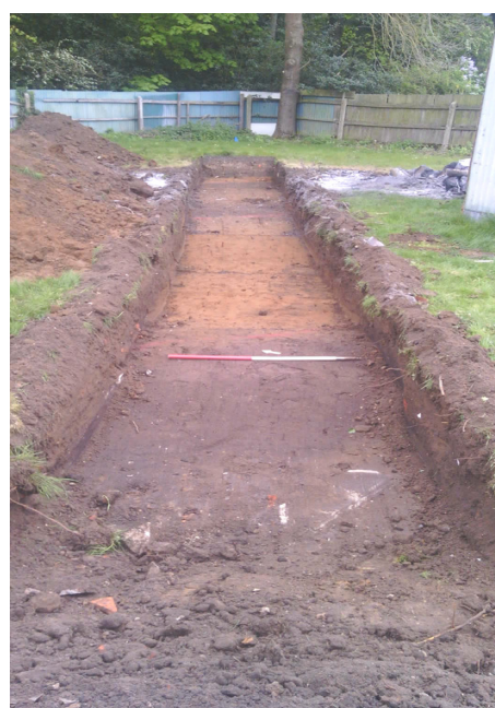
Photograph 2 T2 trench shot – looking northeast
