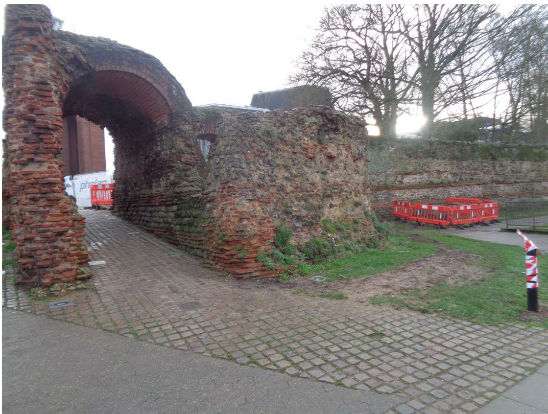
Photograph 9 Photograph showing position of lights around the southern side of Balcerne Gate (after backfilling and reinstatement), looking south-east
