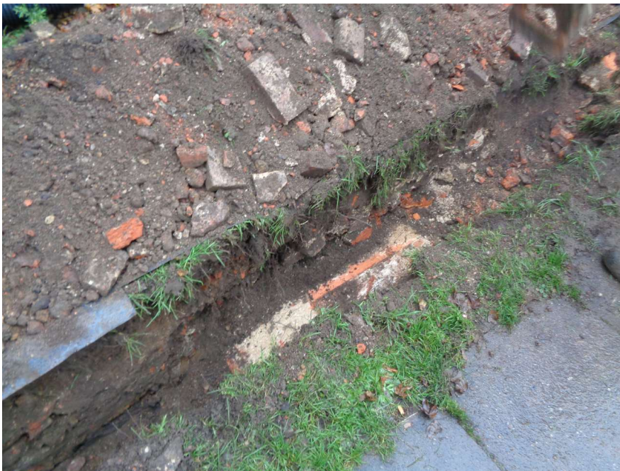
Photograph 11 Brick wall foundation F3, looking southeast
