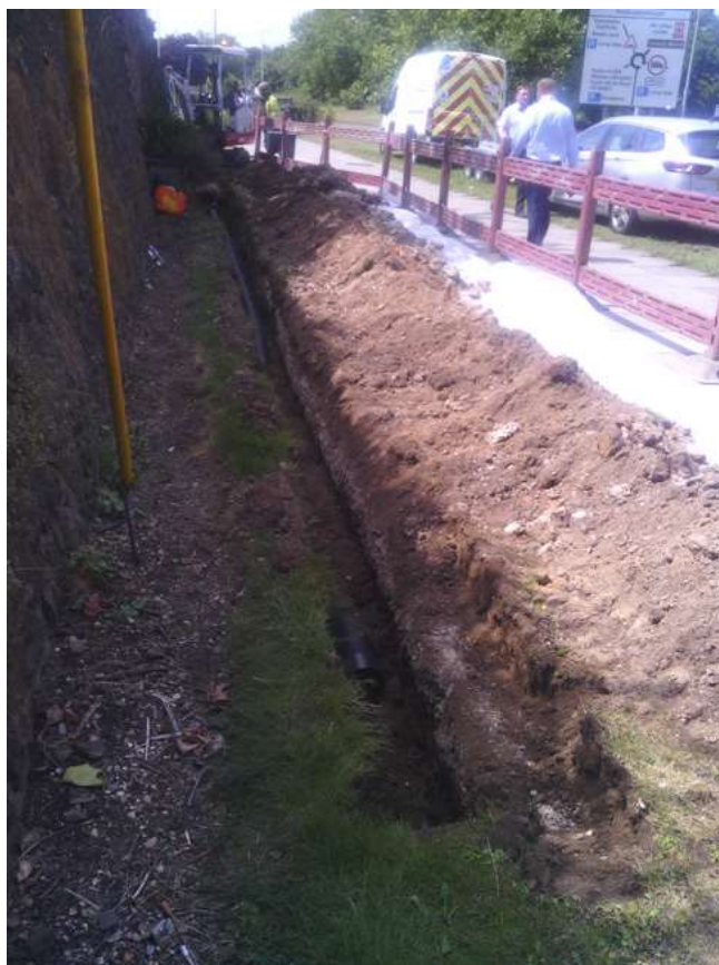
Photograph 3 Phase 1 power cable trench along Middleborough, looking west.
