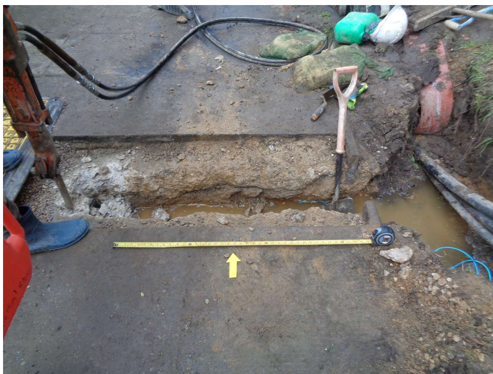
Photograph 8 Phase 2 North of Balkerne Gate – trench across the footpath, looking north.
