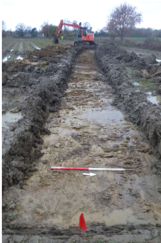
Photograph 15 T458 trench shot – looking west
